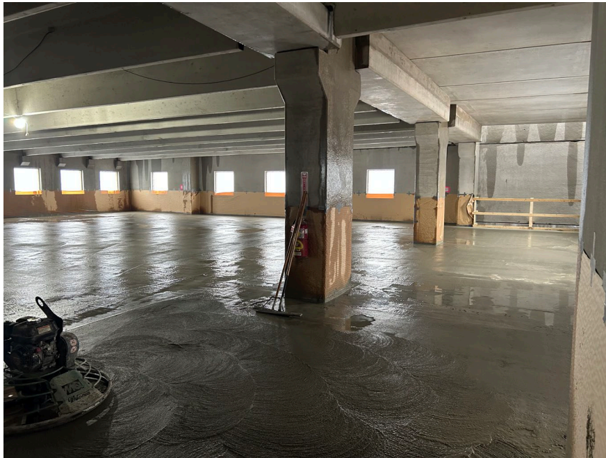
Photo 4: Concrete pouring completed and leveled in office space on floor 2.
