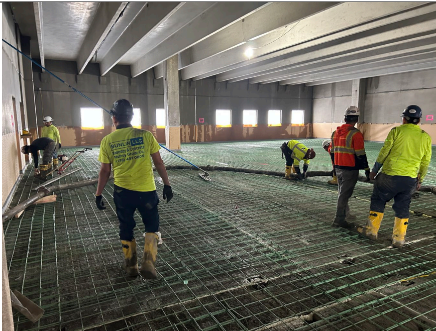
Photo 2: Preparing for concrete pouring in the office space of floor 2.
