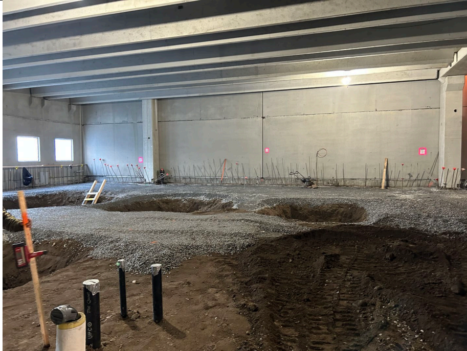
Photo 3: Piles uncovered in A4 and stone placement continues before vapor barrier and SSDS installation.
