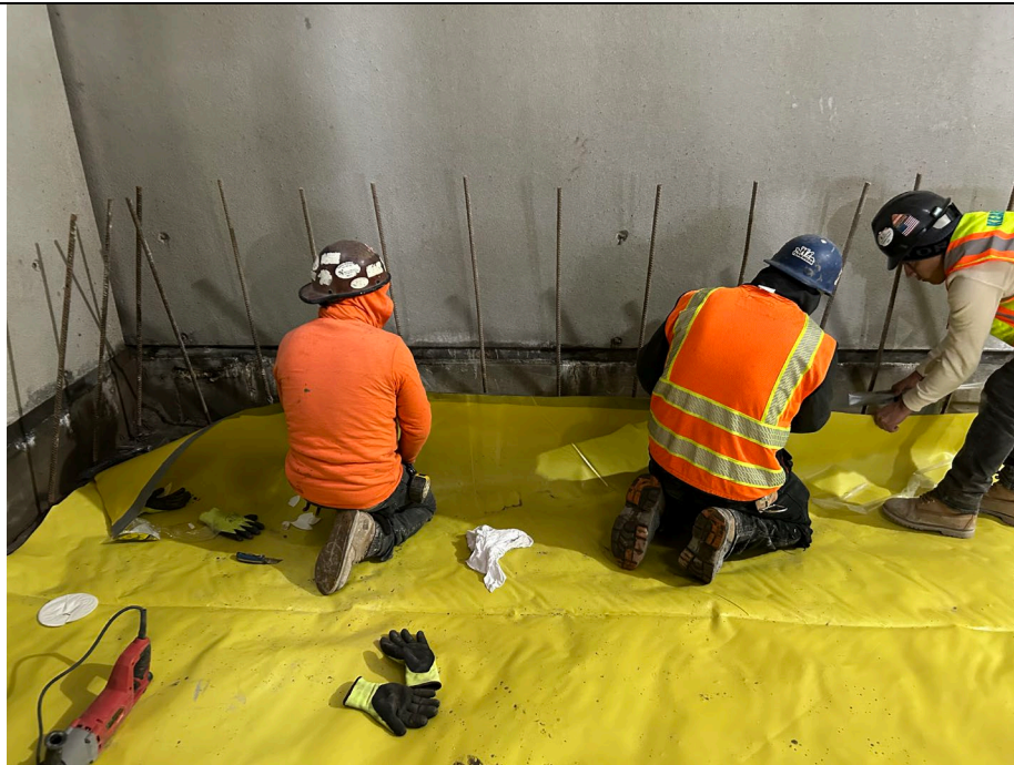
Photo 2: Vapor barrier installation in grid A4.
