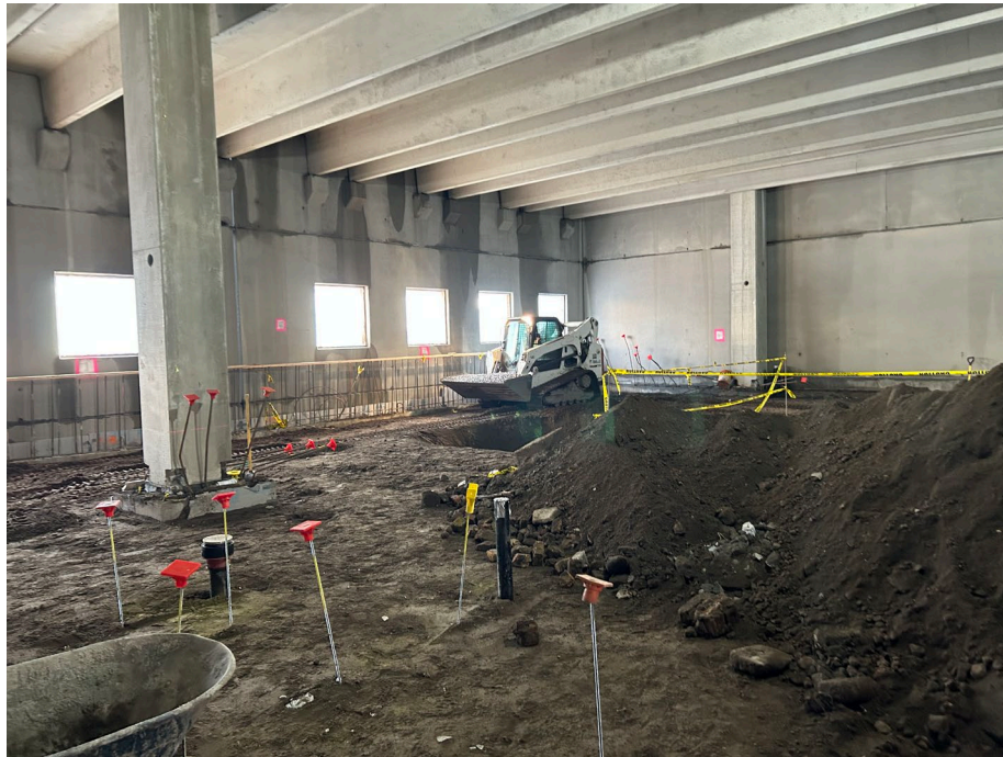
Photo 1: Re-excavation of slab piles in grid A4 and stone placement before vapor barrier and SSDS installation.
