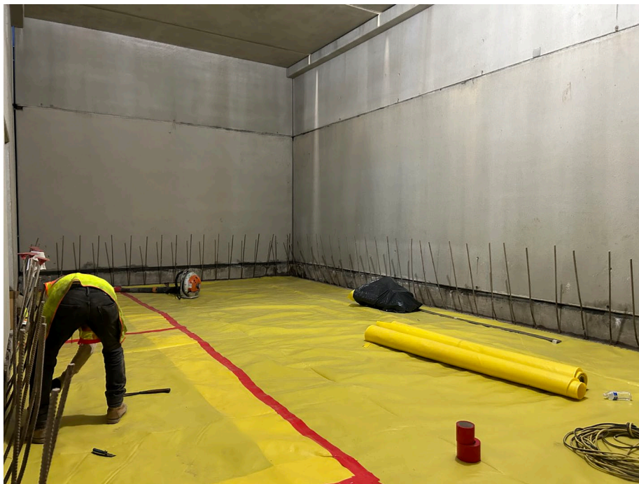
Photo 4: Vapor barrier installation complete in grid A4.
