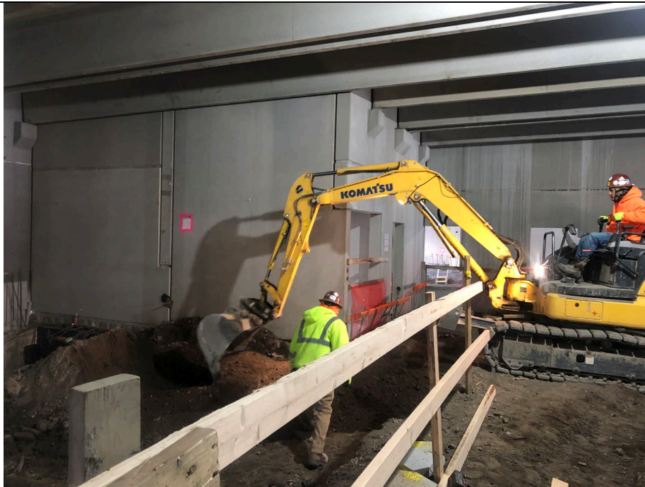
Photo 2: Kingdom backfilling around previously installed plumbing in A3.
