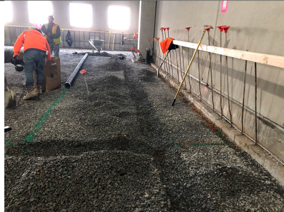
Photo 3: Kingdom began trenching and marking out the layout for SSDS in A4.
