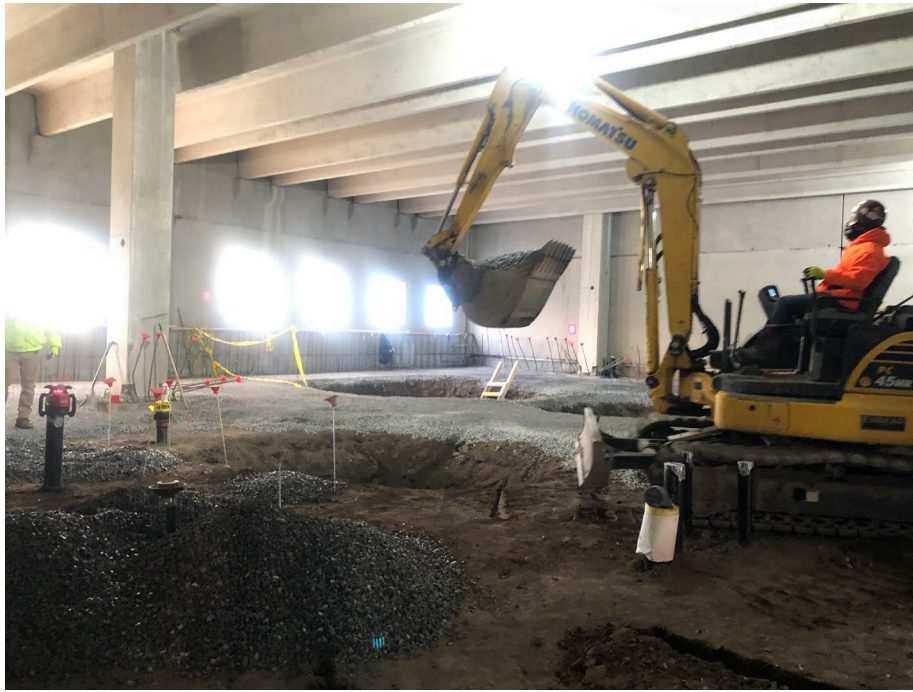
Photo 1: Kingdom continuing to place stone in grid A4.
