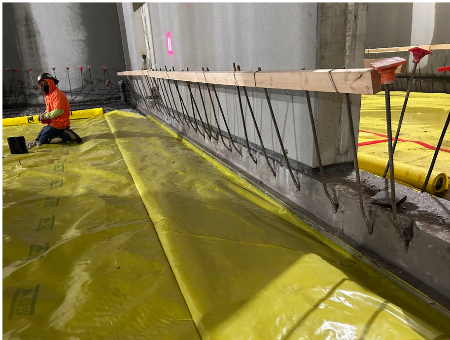
Photo 4: Vapor barrier installation progress in grid A4. Example of termination at concrete wall is in view as installation is being finalized.
