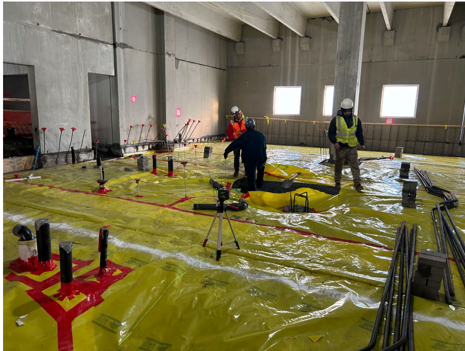
Photo 1: Rebar installation begun and utilities installation was completed in A4. Roux continued to inspect vapor barrier installation.
