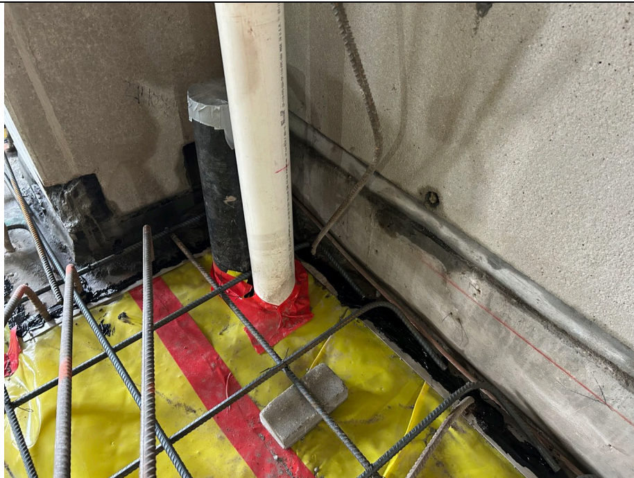
Photo 2: Detail around SSDS riser and utilities pipe. Detail of termination bar as well as tape and mastic sealant, as necessary.
