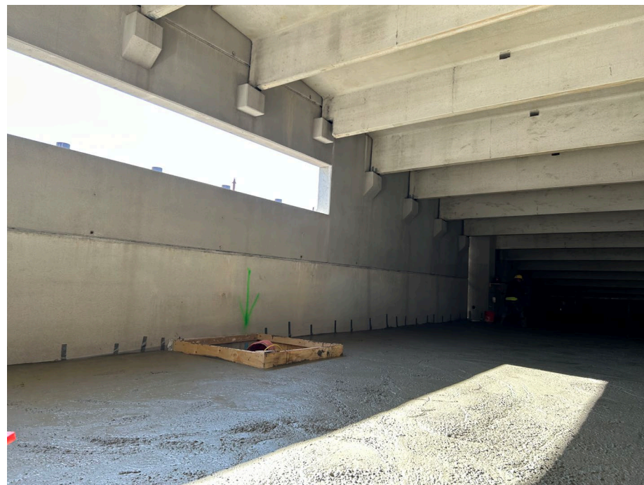
Photo 4: Small area below ramp in B2 boxed out for further utilities installation, vapor barrier to be sealed and inspected after this installation.
