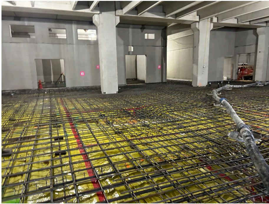
Photo 1: Status of A4 before pouring concrete.
