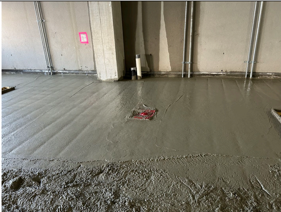
Photo 2: Concrete pour progress on the east end of grid A4. SSDS monitoring point is indicated in red (for protection).
