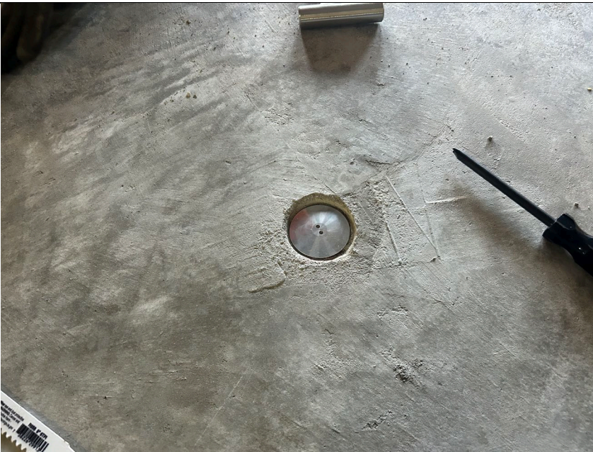
Photo 2: SSDS monitoring points installed, protective metal cap secure on top of vapor pin.
