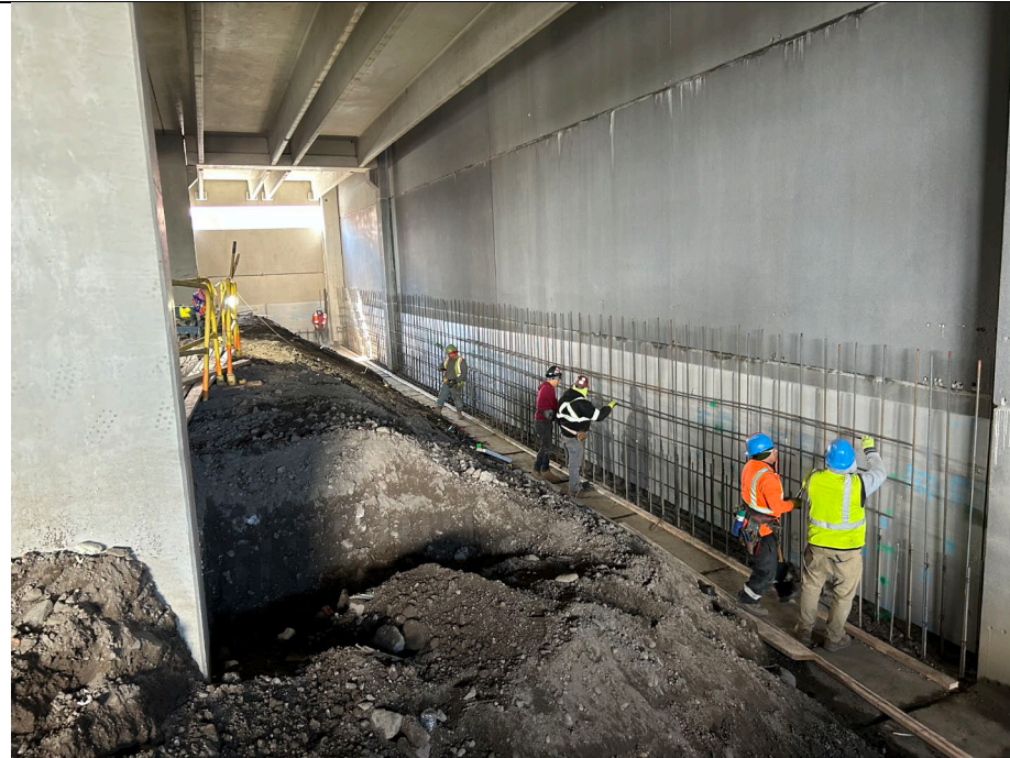
Photo 3: Rebar placement for upcoming concrete pour on western retaining wall.
