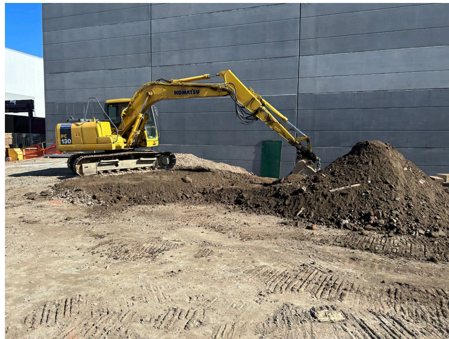
Photo 4: Kingdom moving soil outside of superstructure to accommodate access to foundation elements.
