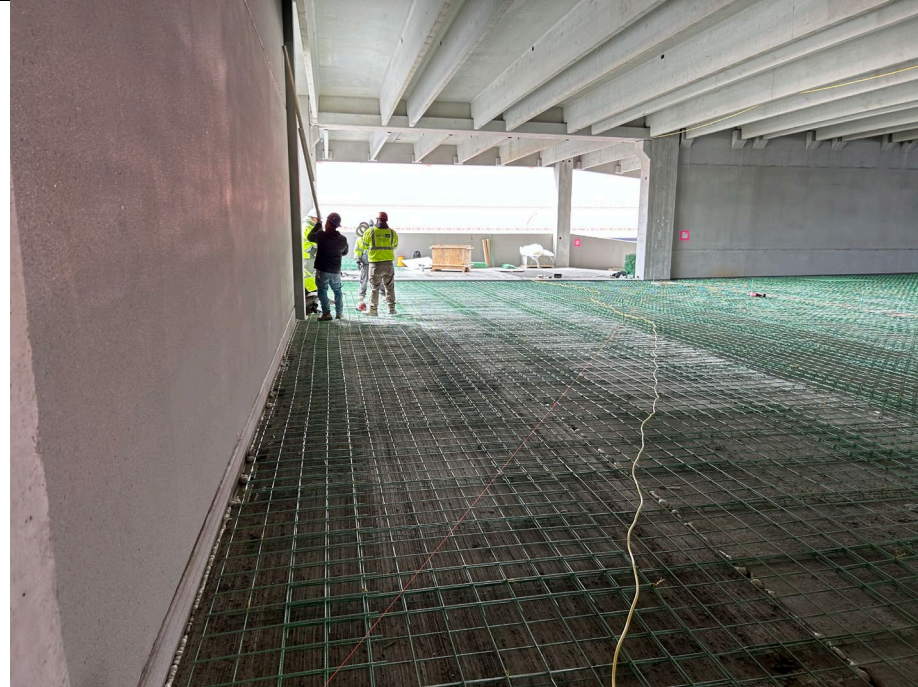
Photo 3: Rebar placement on second floor for nonstructural concrete.
