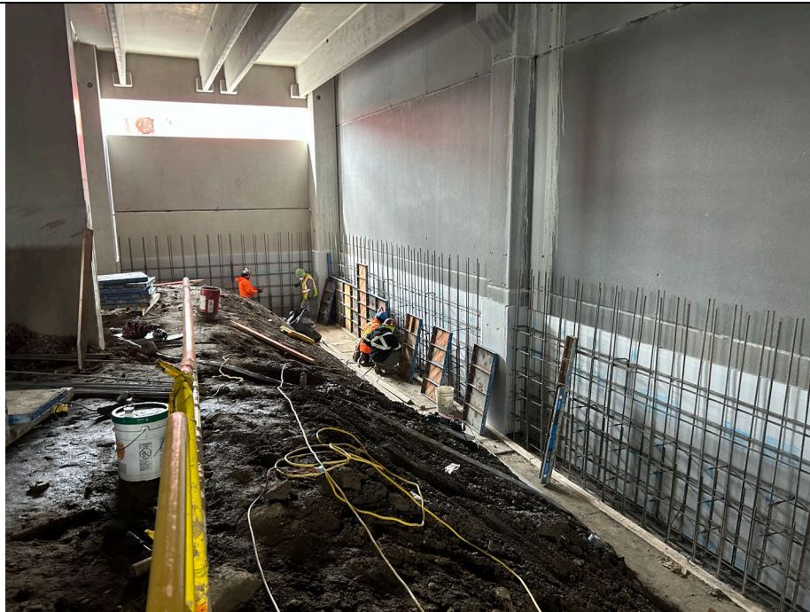
Photo 2: Concrete forms being added to rebar.
