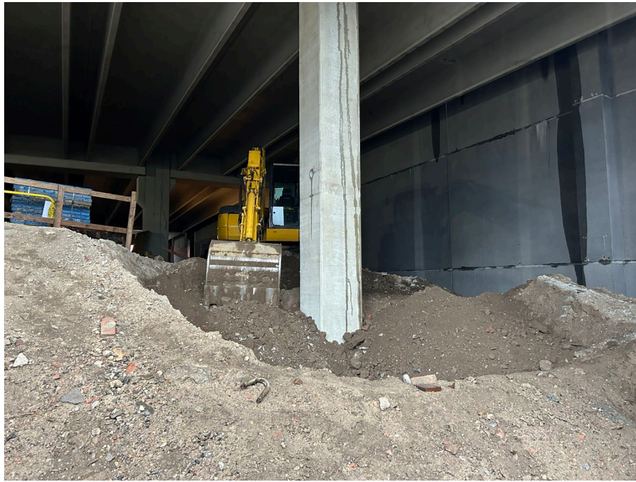
Photo 1: Minor grading around previously laid concrete pile.
