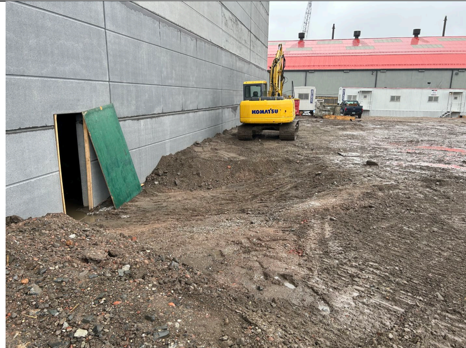
Photo 3: Soil movement outside of superstructure to facilitate access to work area.
