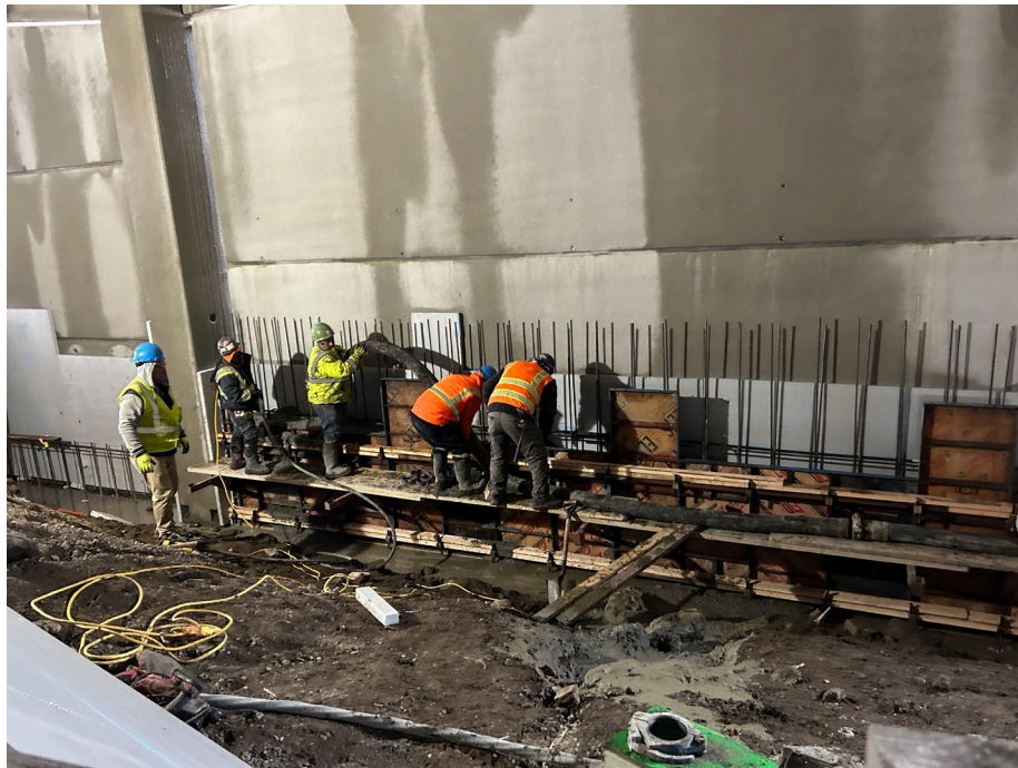
Photo 4: View during concrete pour for retaining wall.
