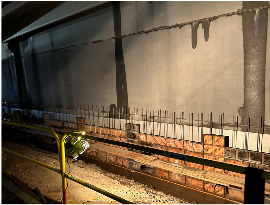
Photo 1: Forms prepared for concrete wall pouring.
