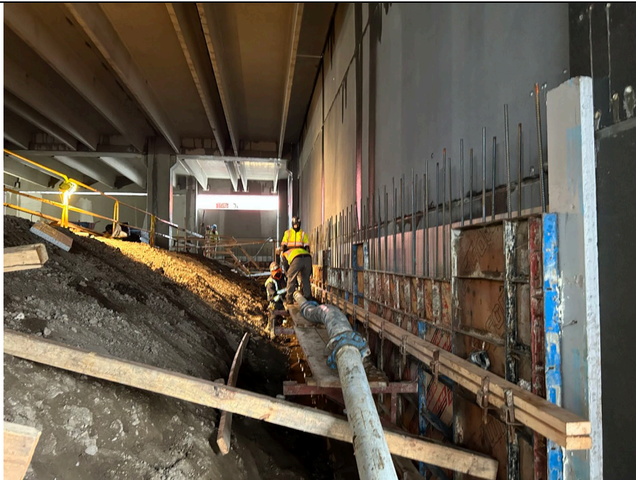
Photo 2: Pump in place and lengths being added before concrete pour begins.
