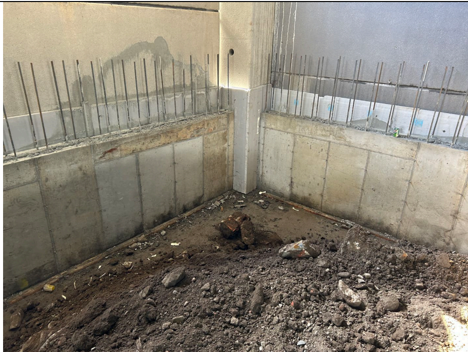
Photo 2: Retaining wall in southwest corner after pour complete.
