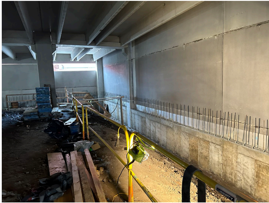
Photo 1: Forms removed from concrete retaining wall.
