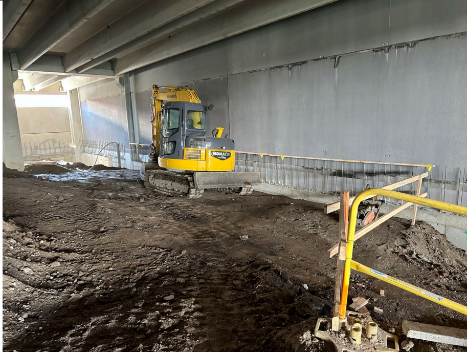
Photo 3: Grading next to retaining wall in B1.
