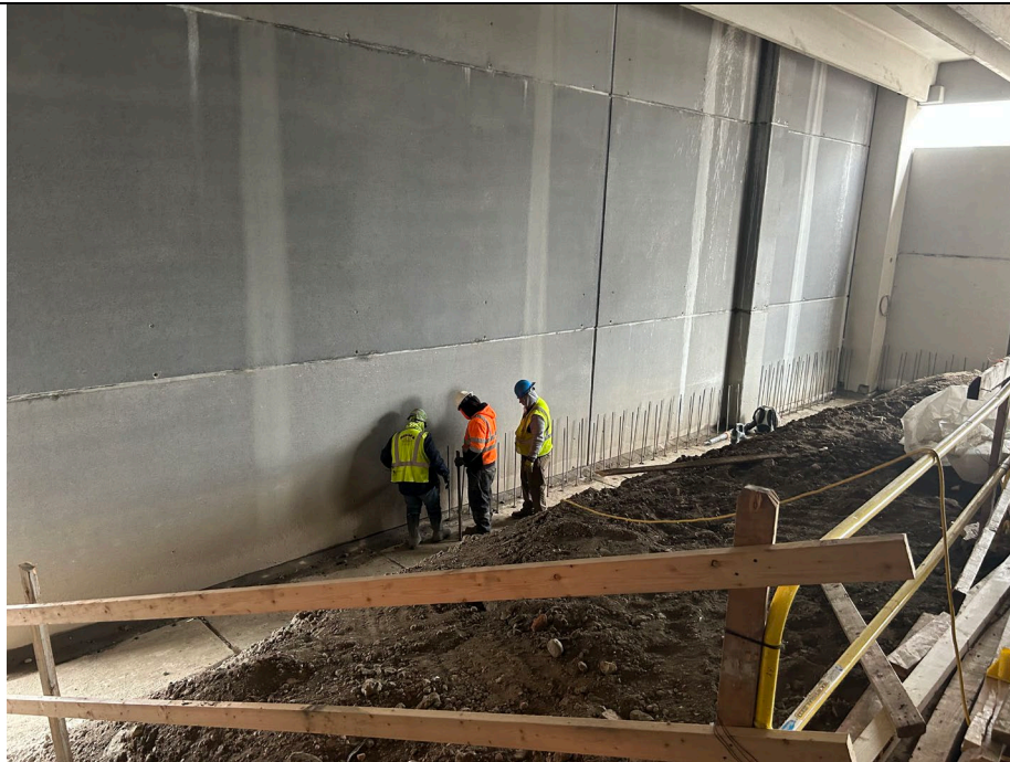
Photo 2: Rebar installation for retaining wall occurring in grid A1.
