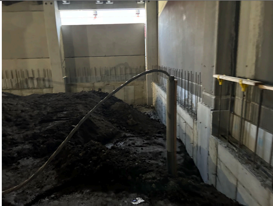
Photo 3: Forms removed from concrete retaining wall and power supply for upper floors wiring was reinstalled.
