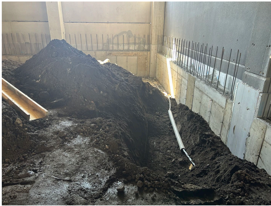
Photo 1: Minor soil movement occurred to re-install electrical wiring in grid B1.
