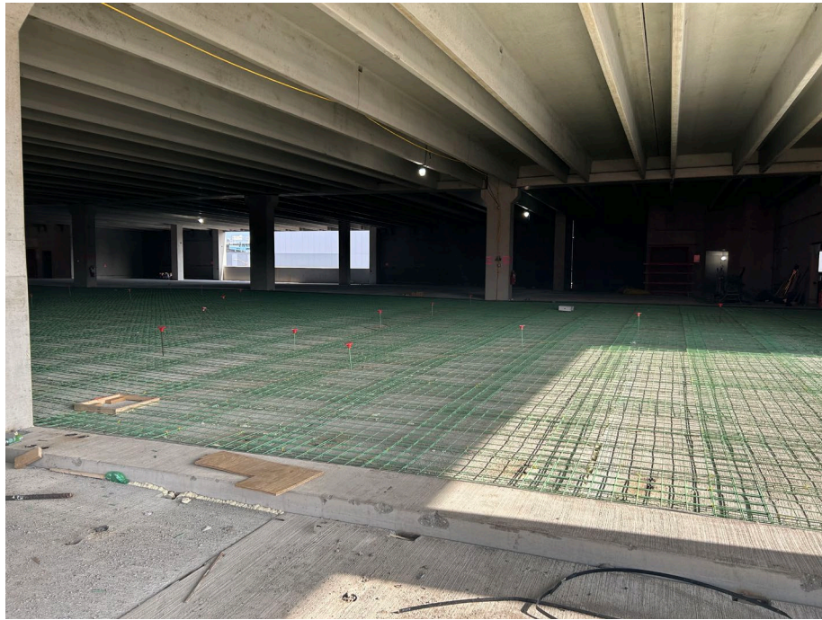
Photo 1: Status of preparation for second floor non-structural concrete pour.
