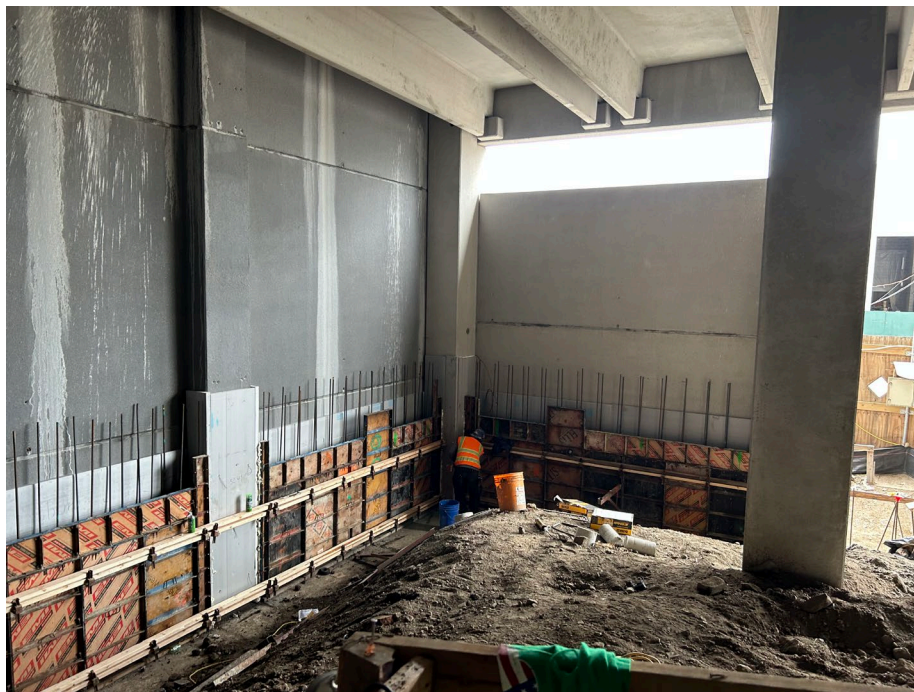
Photo 4: Concrete forms installation in A1.
