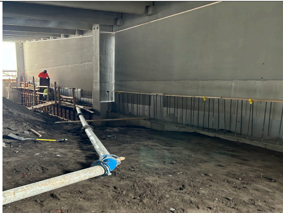
Photo 2: Final forms and rebar installation between B1 and B2, with concrete pump in place for future concrete pour on Monday.
