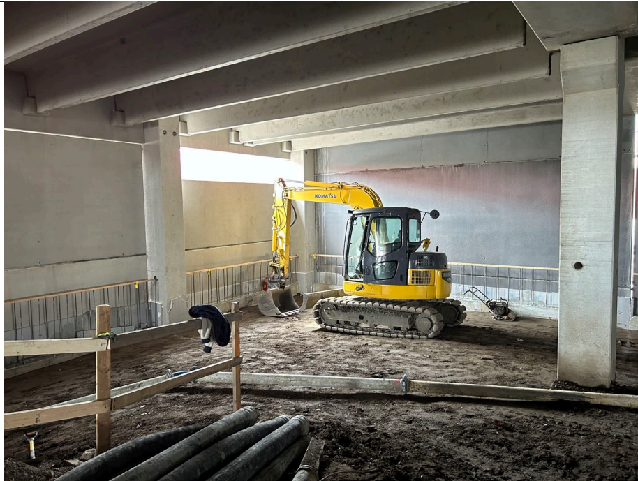
Photo 3: Grading around retaining walls in grid B1.
