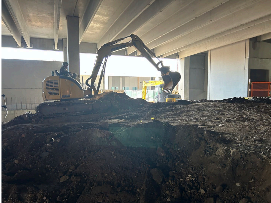
Photo 3: Soil movement in A1 to prepare for soil export and backfill around retaining wall poured yesterday.
