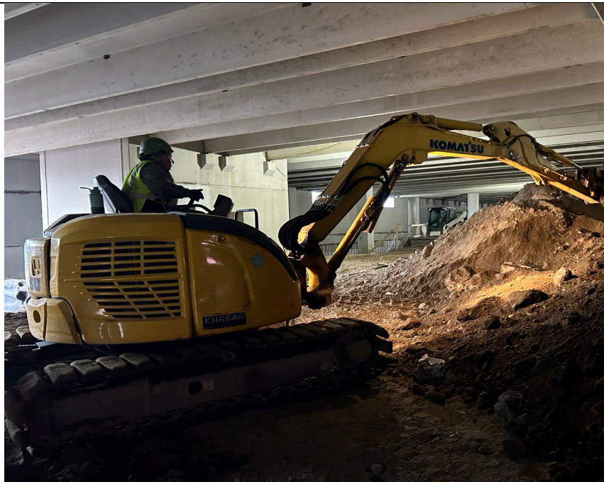
Photo 2: Preparing material for export from under superstructure.
