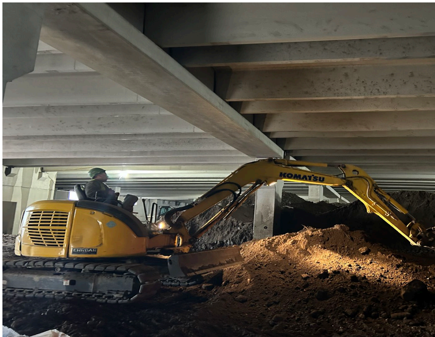
Photo 4: Progress of preparing material for export from under superstructure.
