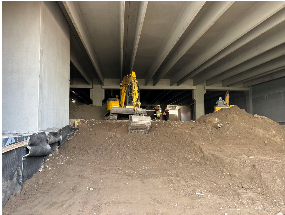
Photo 1: Kingdom managing soil ramp in A1 leading from inside of the building to prepare for export.
