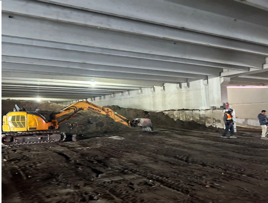
Photo 3: Status of soil movement from under superstructure at end of the day.
