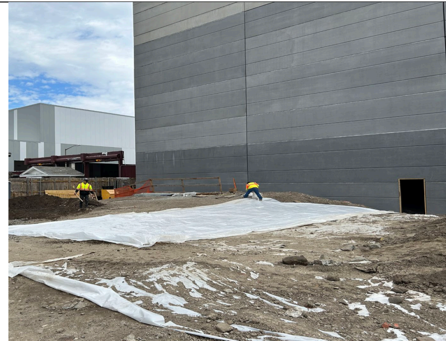
Photo 2: Contractors adding another layer of poly sheeting in temporary storage area before placing additional material.
