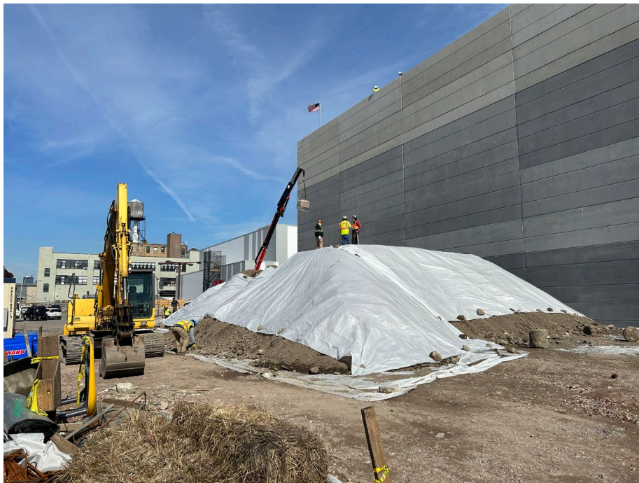
Photo 4: Covering of stockpile with poly sheeting at the end of the day.
