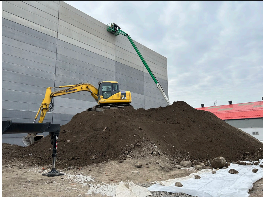
Photo 3: Consolidation of material outside of superstructure in preparation for offsite disposal continues.
