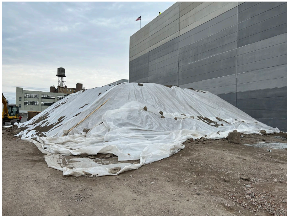
Photo 4: Temporary stockpile was covered at the end of the workday.
