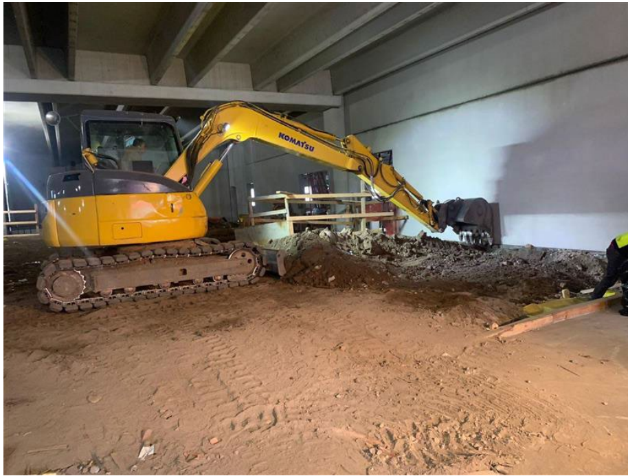
Photo 1: Kingdom begins grading soil in grid B3 along walls.
