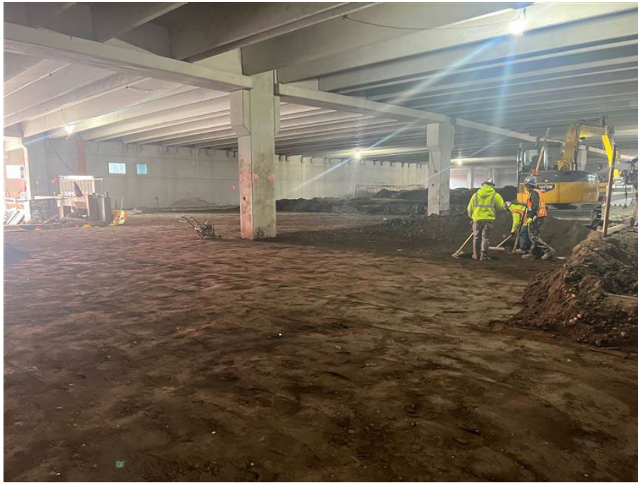
Photo 1: Progress made by grading soil in grid A3.
