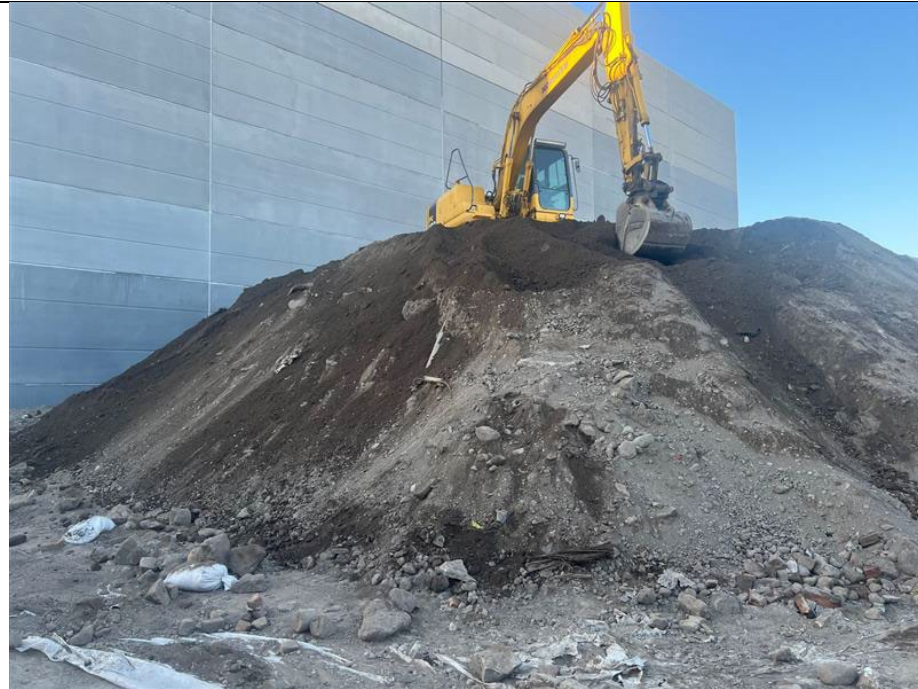
Photo 3: Kingdom consolidates material outside of superstructure in preparation for offsite disposal continues.
