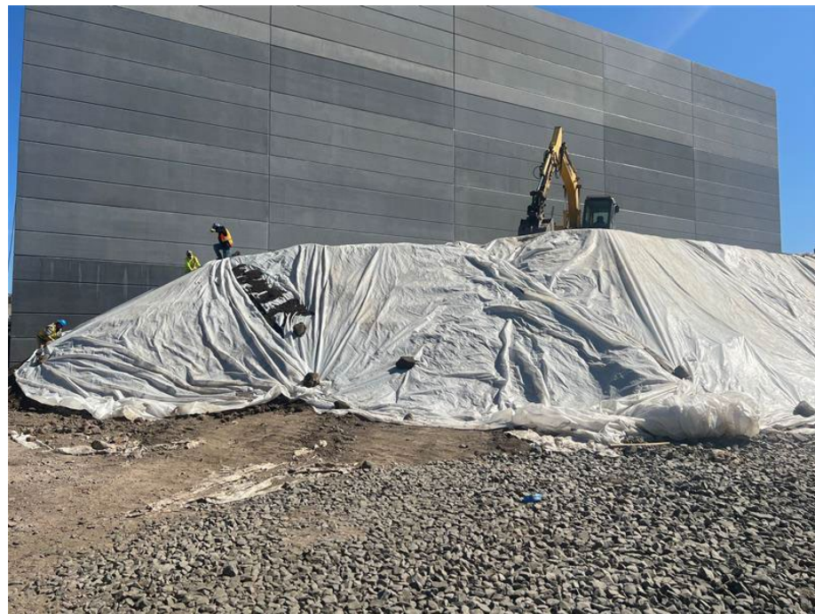
Photo 4: Temporary stockpile covered at the end of workday.
