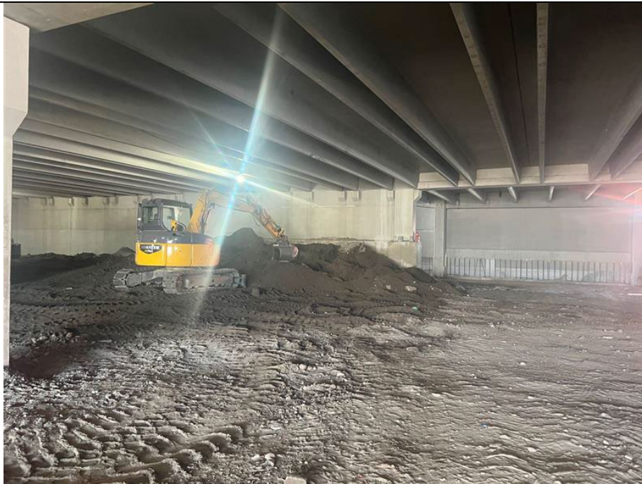
Photo 2: Status of excess soil on the ground floor within the building in grid B1.
