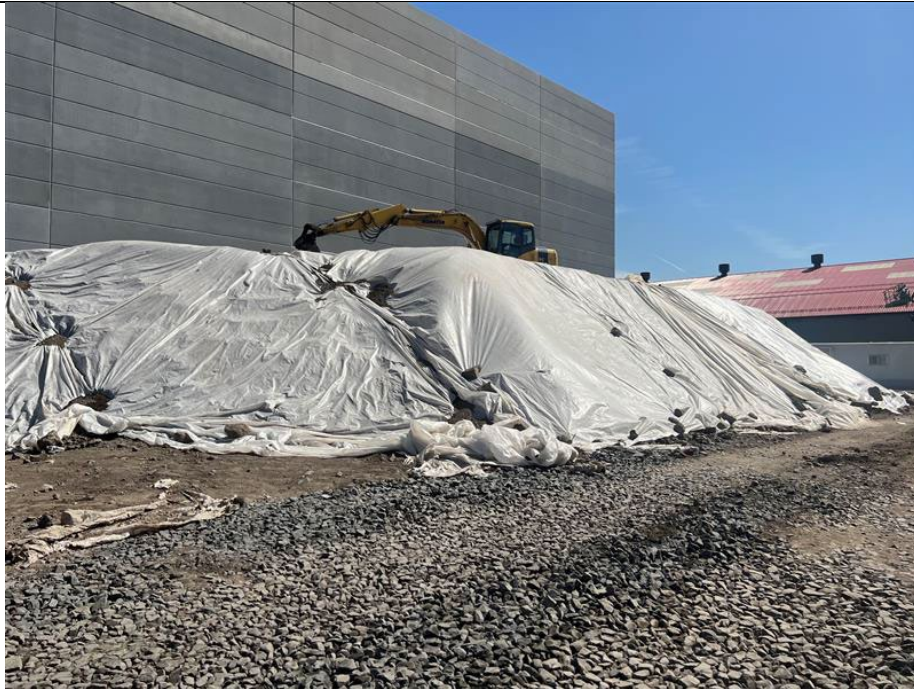
Photo 3: Temporary stockpile covered at the end of workday.
