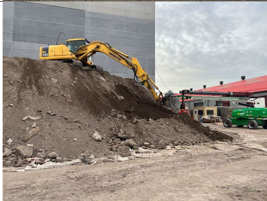
Photo 2: Kingdom performing maintenance on temporary stockpile outside superstructure.
