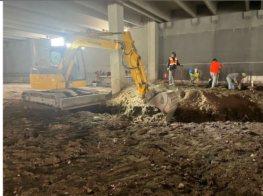
Photo 3: Kingdom excavating in grid A2 and A3 for additional utilities installation.
