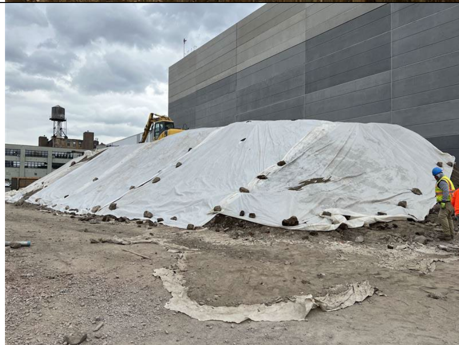
Photo 4: Temporary stockpile covered and secured at the end of workday.
