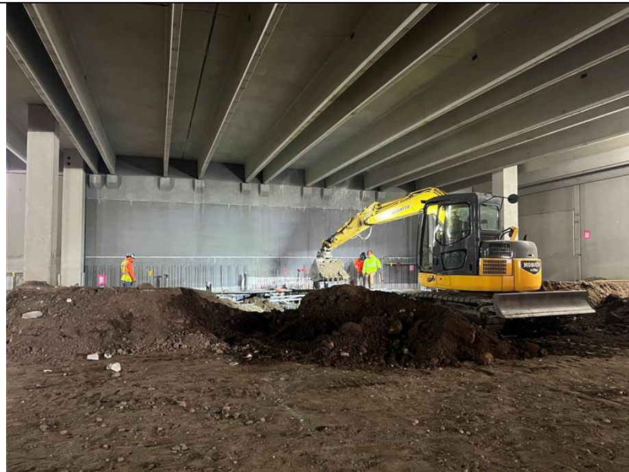
Photo 1: Looking east, kingdom backfilling around completed utilities in grid A3.
