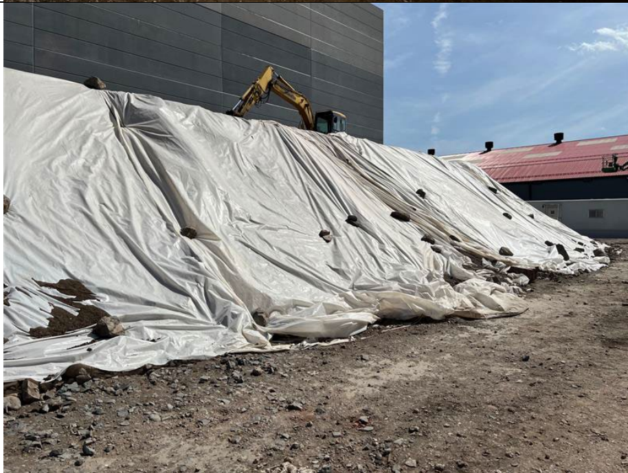
Photo 4: Temporary stockpile remained covered throughout workday.
