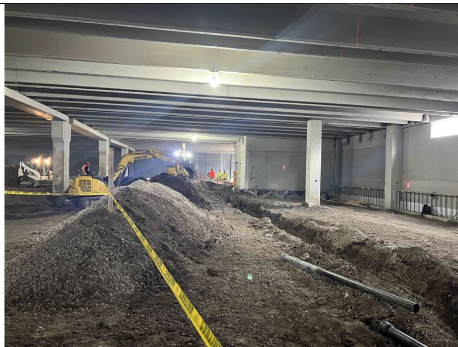
Photo 2: Looking North, Kingdom excavating in grid A1 and A2 for additional utilities installation.
