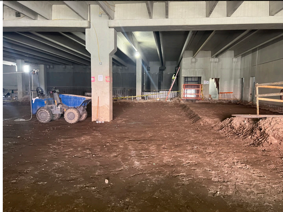
Photo 2: Looking north, Kingdom continues grading soil in A3/B3.
