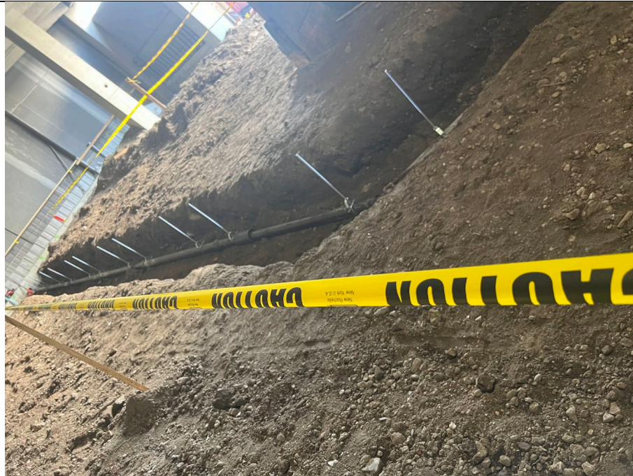
Photo 3: Looking west, plumbing continues within trench.
