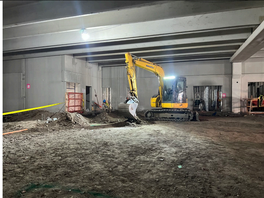
Photo 1: Looking southeast, kingdom continues grading soil in A3.
