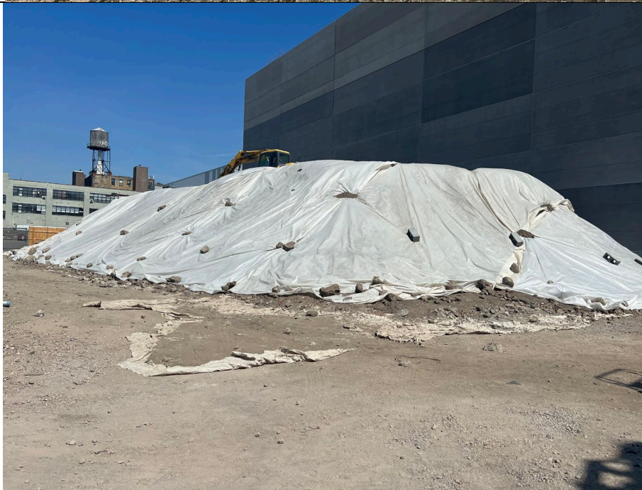
Photo 4: Temporary stockpile remained covered throughout workday.
