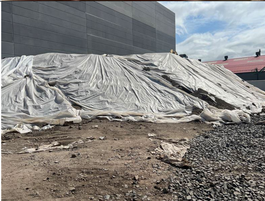
Photo 4: Temporary stockpile remained covered throughout workday.
