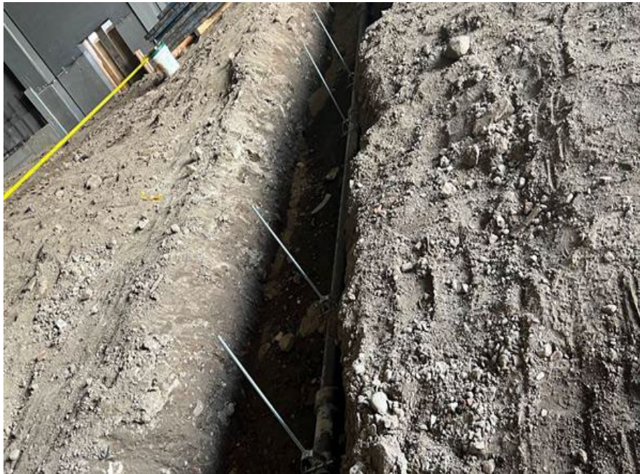
Photo 4: View of plumbing installation within shallow trench.
