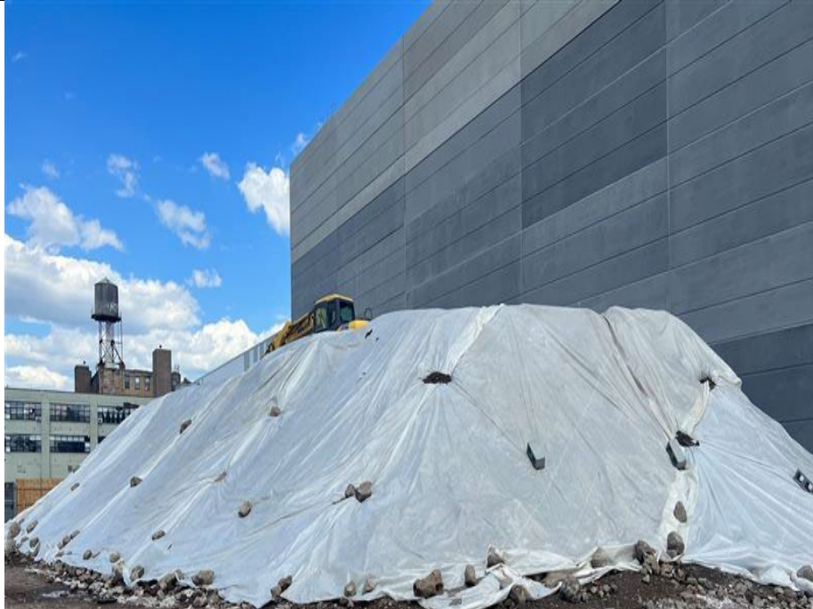
Photo 3: Temporary stockpile remained covered throughout workday.
