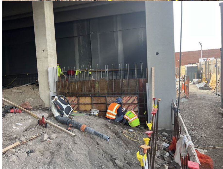
Photo 2: Looking northeast, kingdom adds forms and continues working on wall.
