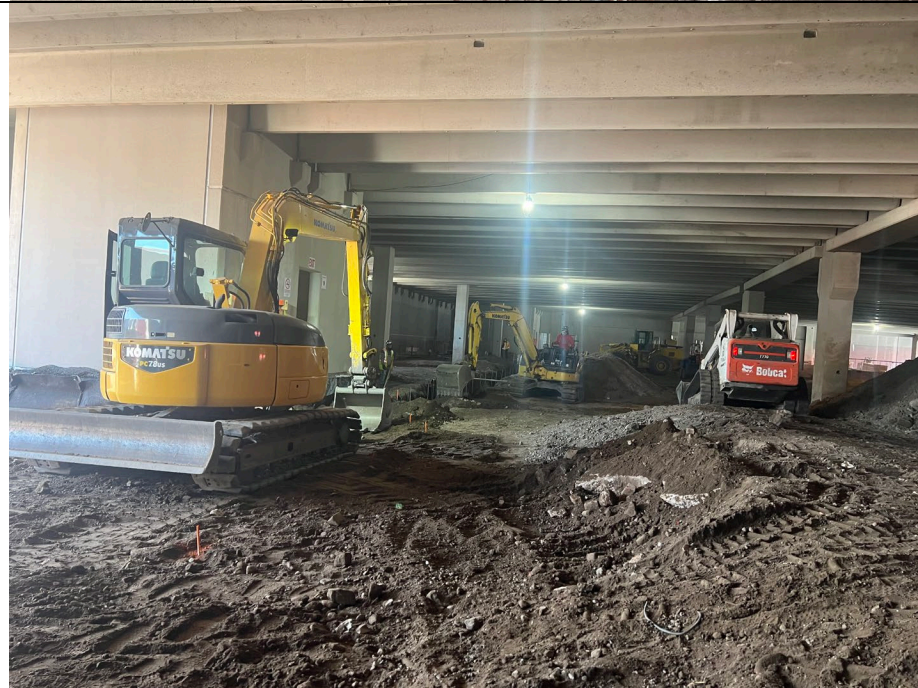
Photo 2: Looking south, kingdom backfilling trench along grids A1 and A3.
