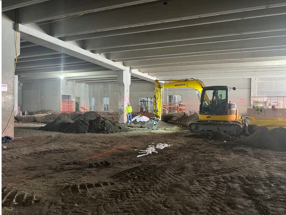
Photo 3: Looking southeast, kingdom excavates in A3 for storm drain installation.
