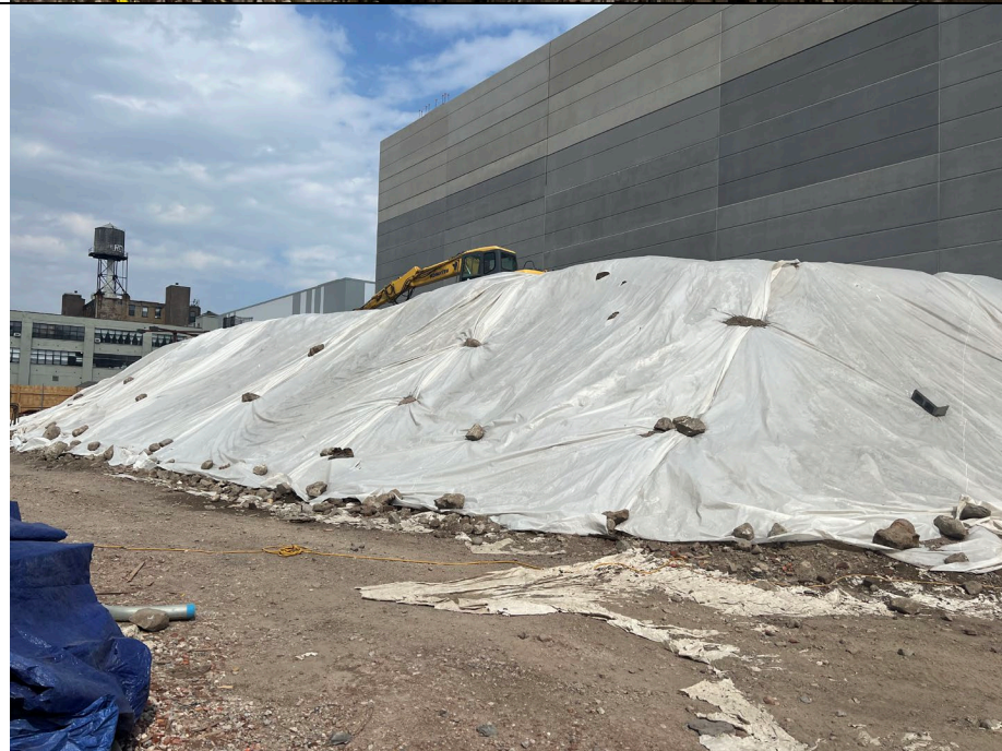
Photo 4: Temporary stockpile remained covered throughout workday.
