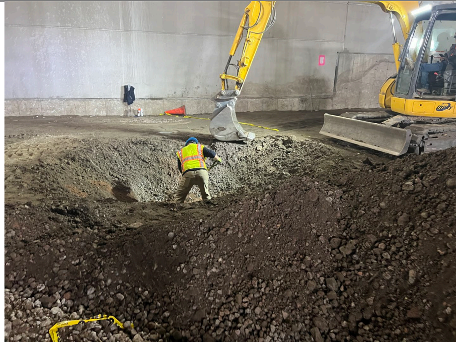
Photo 3: Looking west, kingdom excavates in B2 for pile caps.
