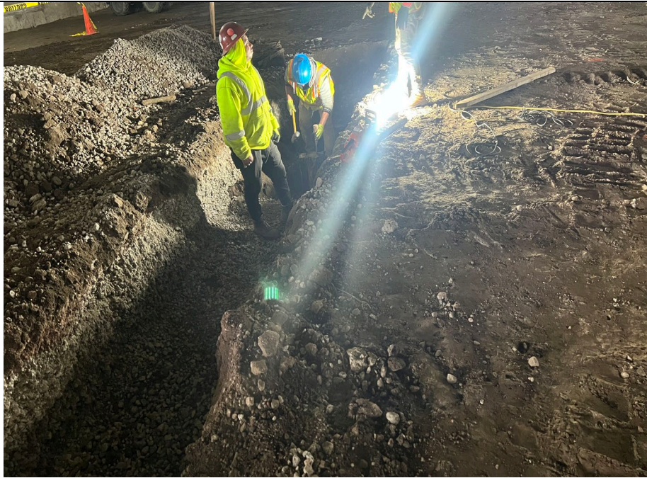
Photo 1: Looking northwest, installation of storm drain in Grids A3 and B3
