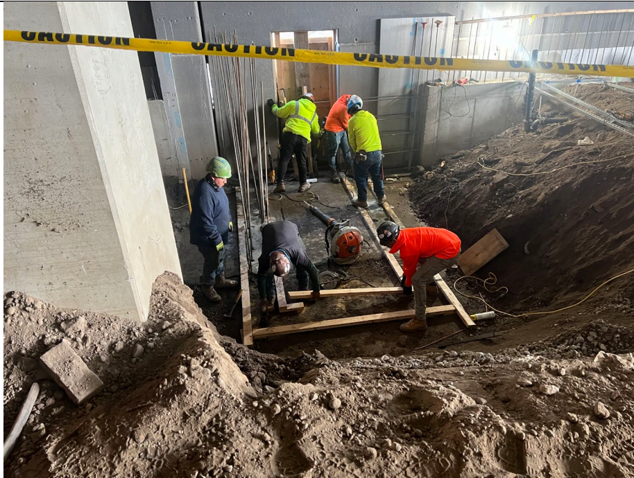
Photo 2: Looking north, Kingdom installing rebar for additional above ground wall.
