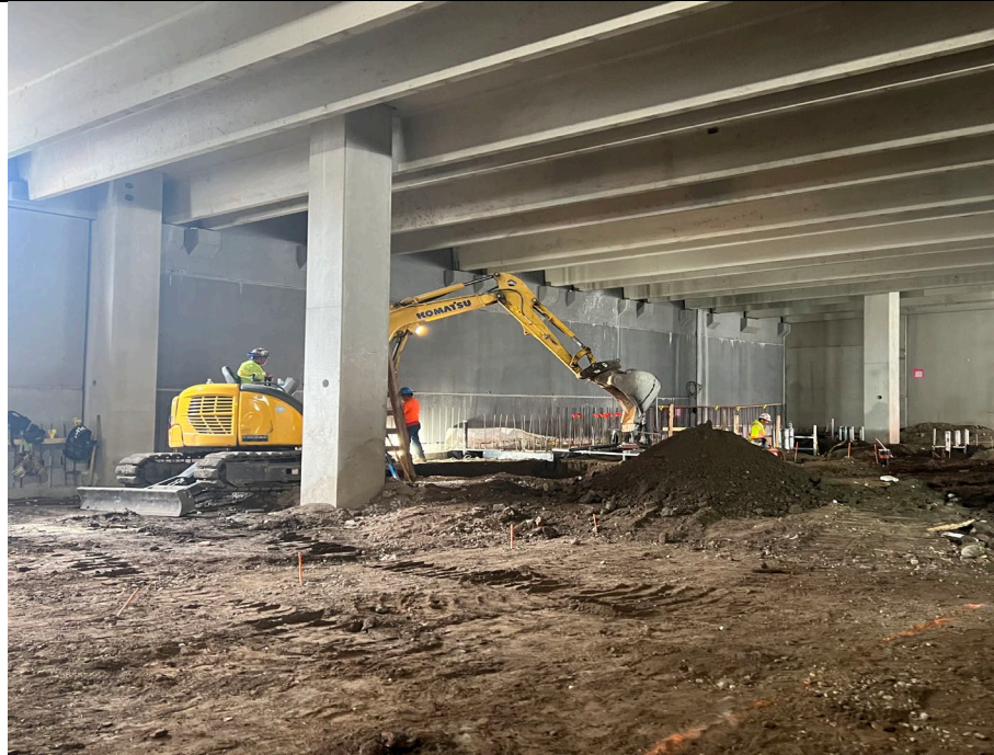
Photo 1: Looking southeast, Kingdom removing portion of previously backfilled material in A3 to allow for utilities modification.
