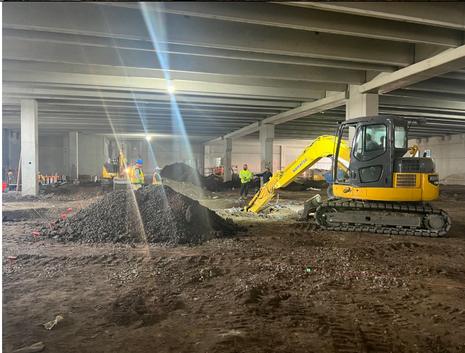
Photo 2: Looking south, Kingdom excavates in A2 for pile caps.
