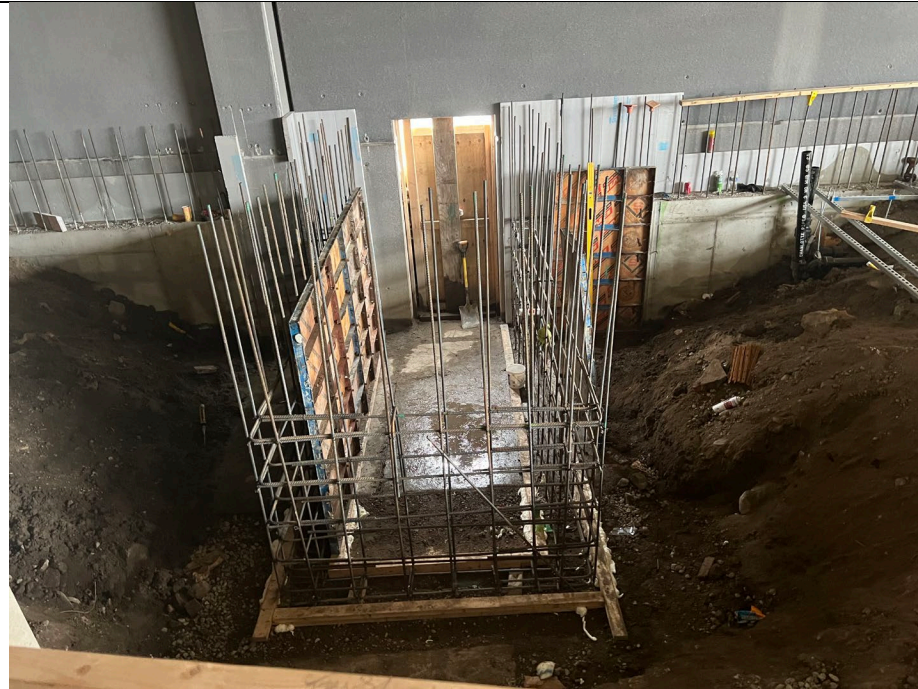
Photo 3: Looking north, kingdom installing rebar and forms for additional wall in A1.
