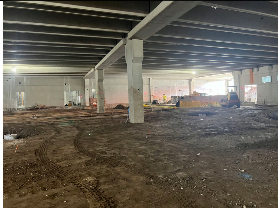
Photo 3: Looking southwest, Kingdom graded material in grid A3 and B3 in preparation for foundation installation.
