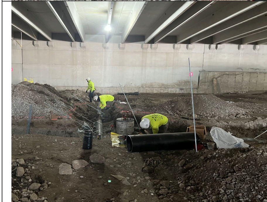
Photo 2: Looking west, storm drainpipe installation continues in B2.
