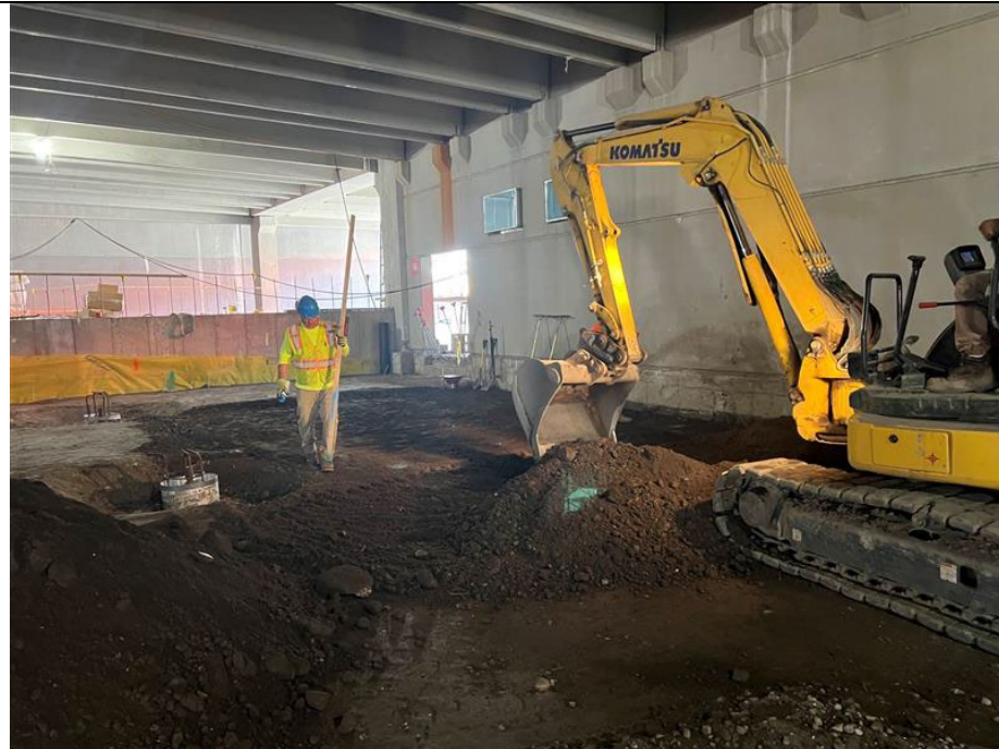
Photo 1: Looking southwest, kingdom grading soil in grid B3.
