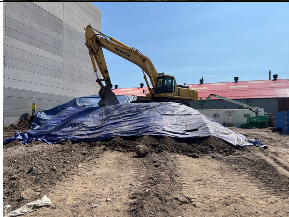
Photo 4: Temporary stockpile covered before the end of workday.
