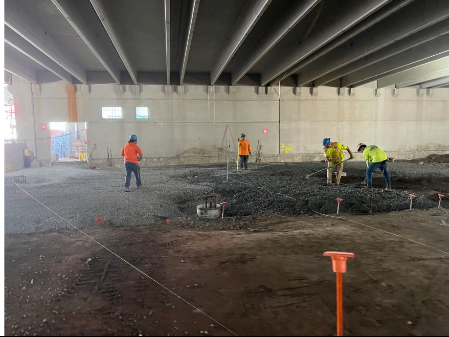
Photo 1: Looking west, kingdom backfilling grid B3 and B2 with \frac{3}{4} " stone.
