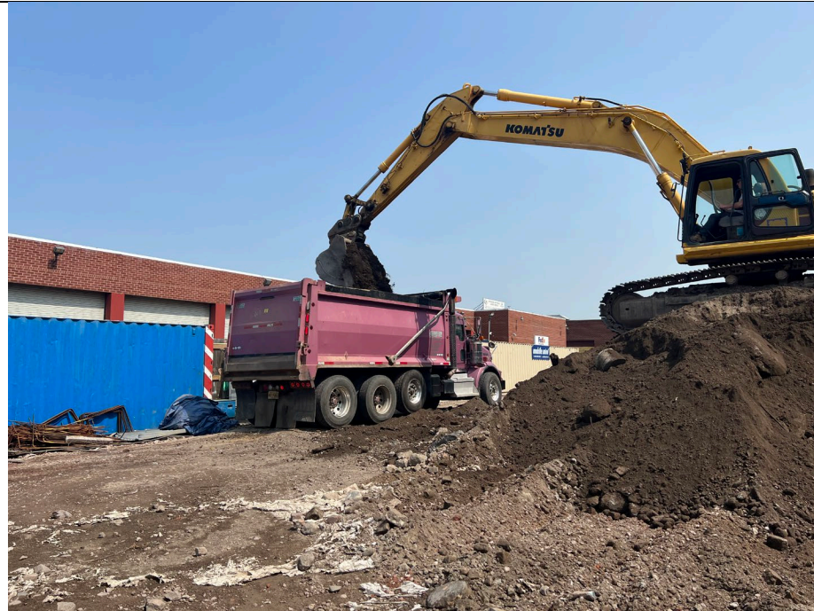
Photo 3: View of truck being loaded with soil for disposal.
