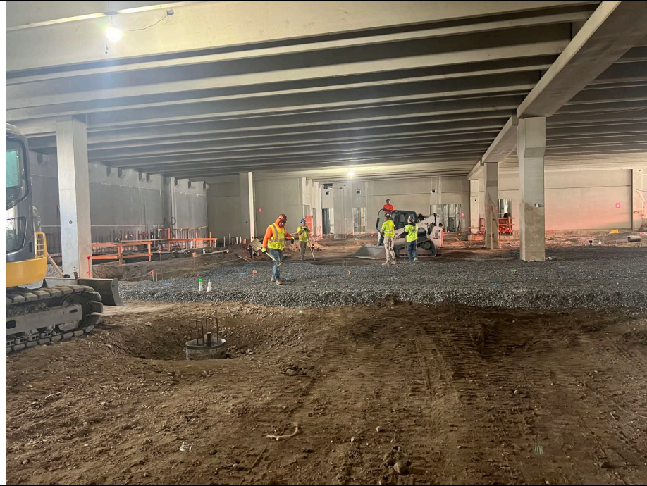
Photo 2: Looking north, stone backfill progress in B2 and B3.
