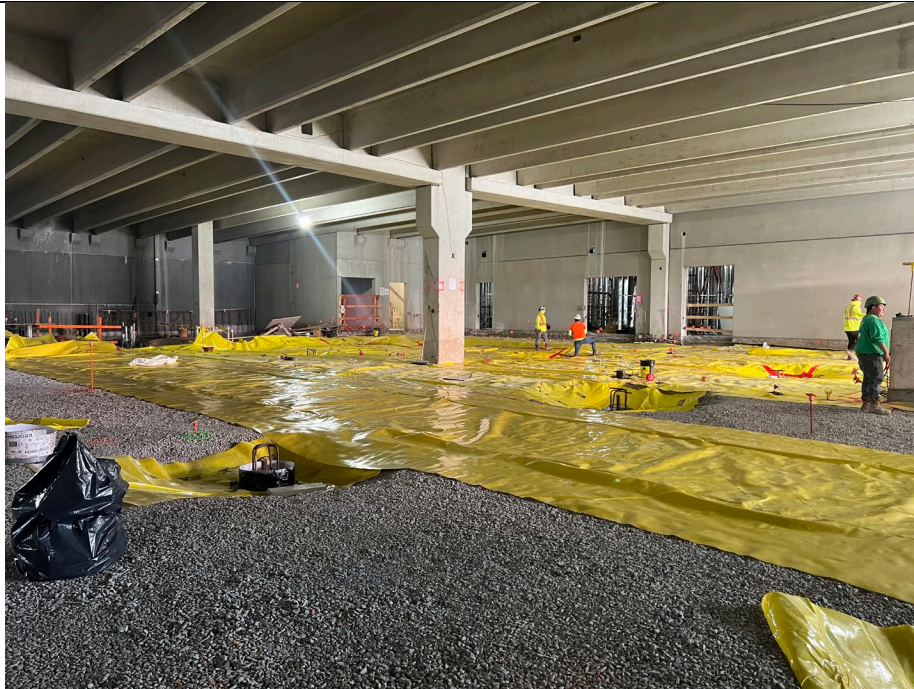
Photo 3: Looking southeast, progress of vapor barrier installation in B3 and A3.
