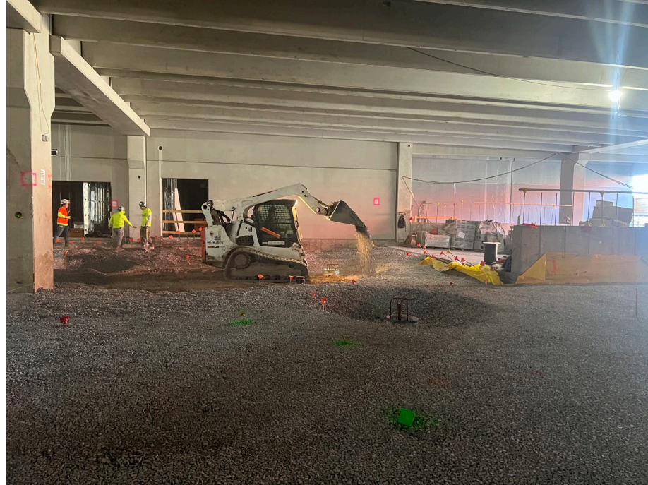
Photo 1: Looking southwest, kingdom backfilling with \frac{3}{4} " stone in grid B3.
