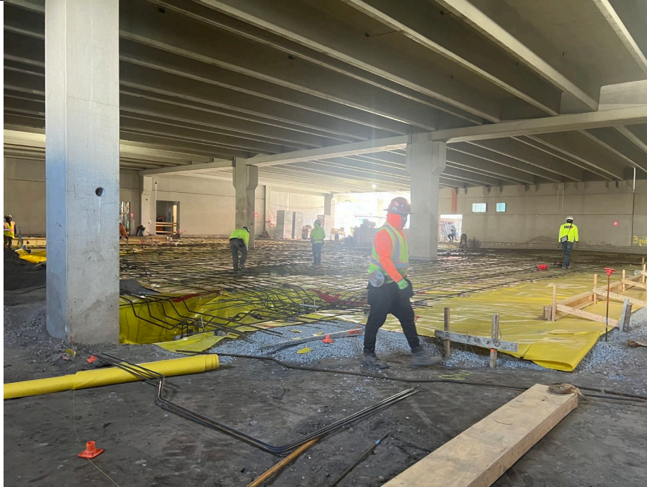
Photo 3: Looking southwest, progress of rebar placement in grid B3-B2 and A3-A2.
