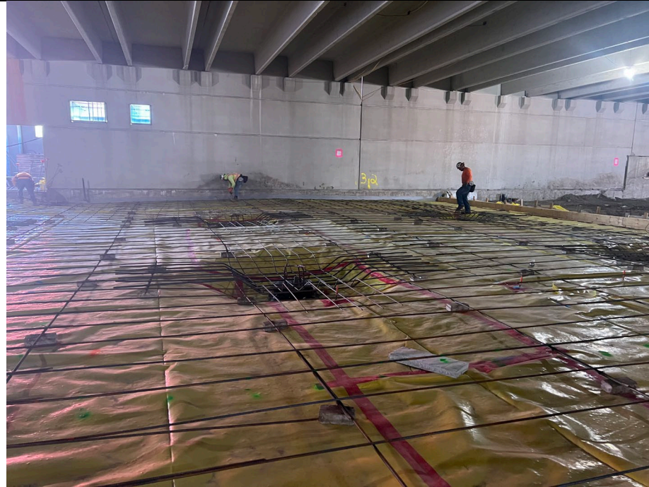
Photo 1: Looking west, kingdom continues rebar installation in preparation for concrete pour.
