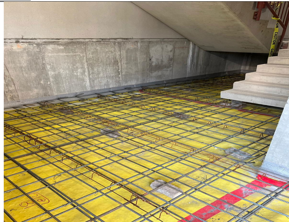
Photo 1: View of rebar placed in staircase A landing in preparation for concrete pour.
