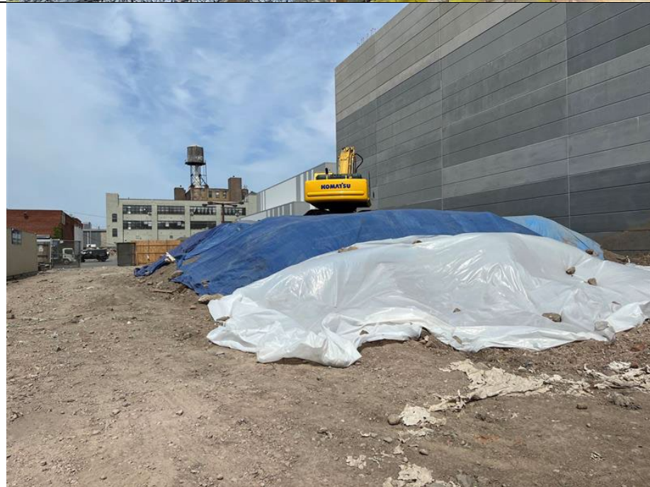
Photo 4: Temporary stockpile remained covered throughout the workday.
