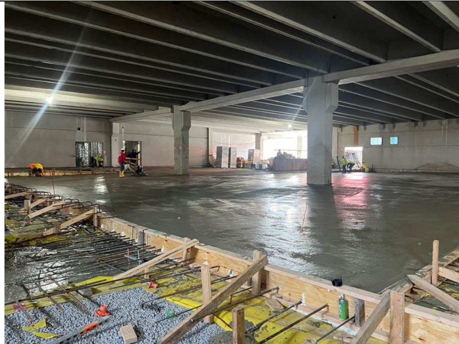
Photo 3: Looking southwest, progress of poured concrete slab.
