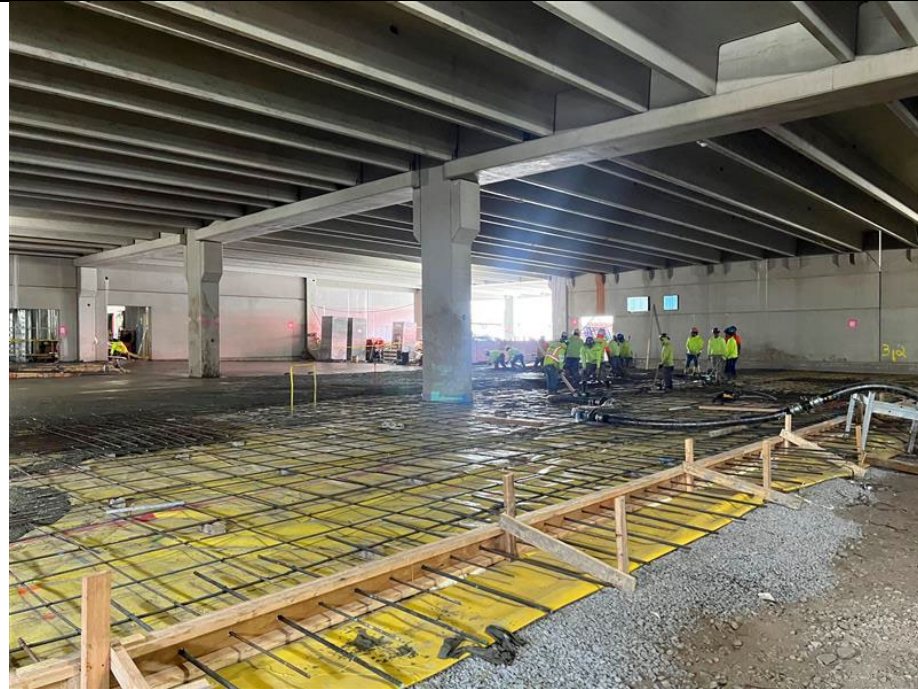
Photo 1: Looking southwest, Kingdom pouring concrete slab in grids B3-B2 and A3-A2.
