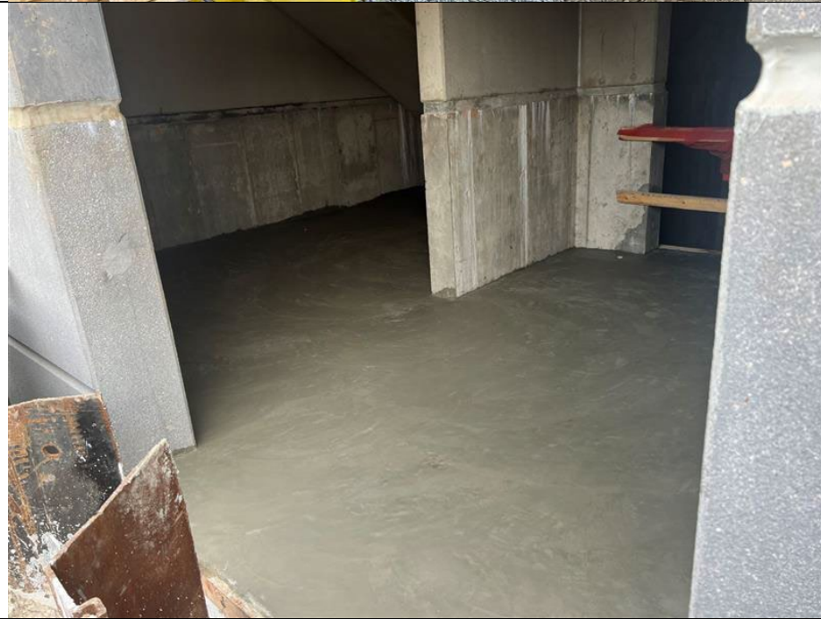
Photo 2: View of poured re-slab in staircase A landing.
