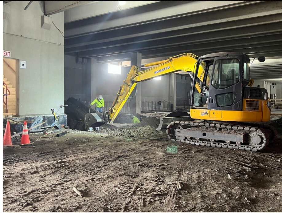
Photo 2: Looking east, view of kingdom excavating trench for storm drain.
