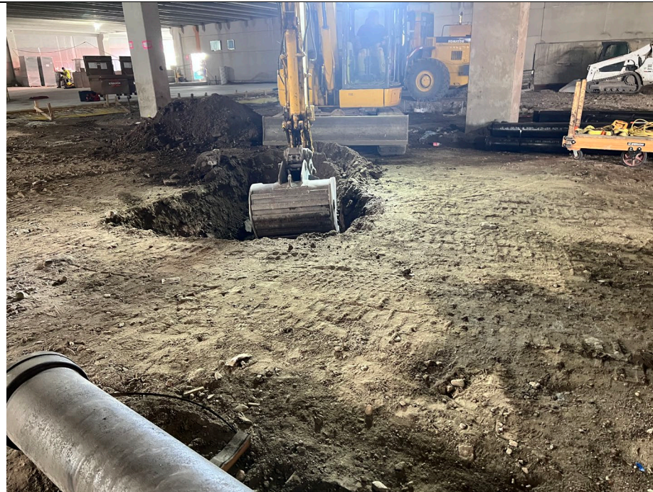
Photo 1: Looking west, Kingdom excavates for pile caps in grid A2.
