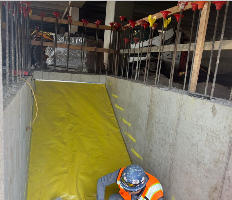
Photo 2: Looking south, view of vapor barrier installation in NW corner of grid A1.
