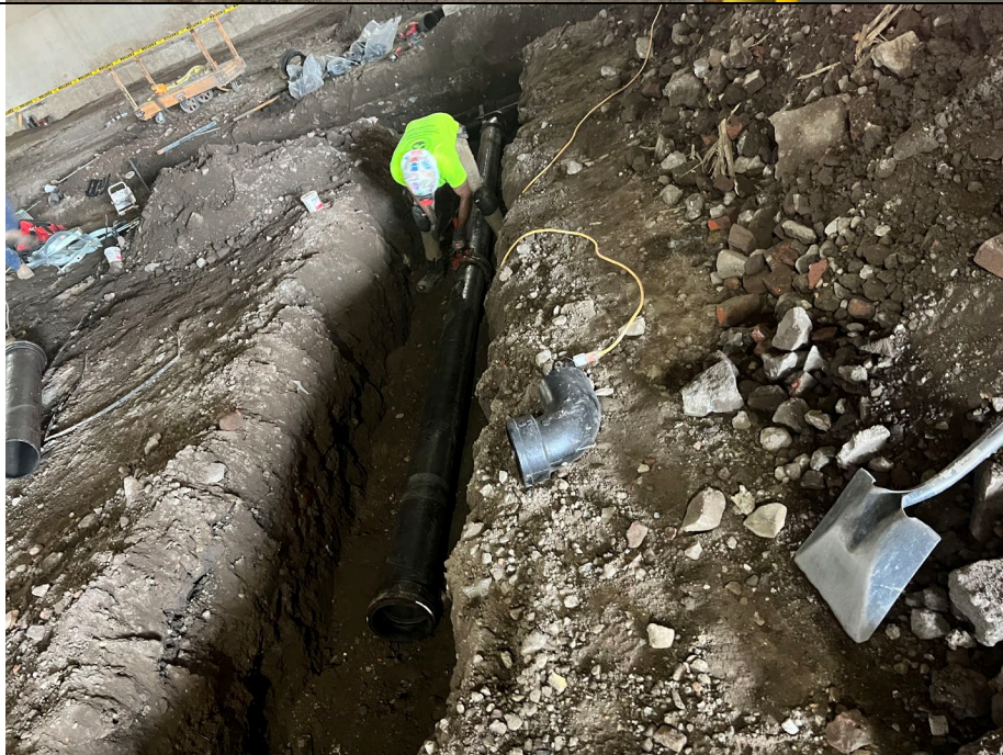
Photo 4: Looking west, view of kingdom continuing storm drain installation in grid B1.
