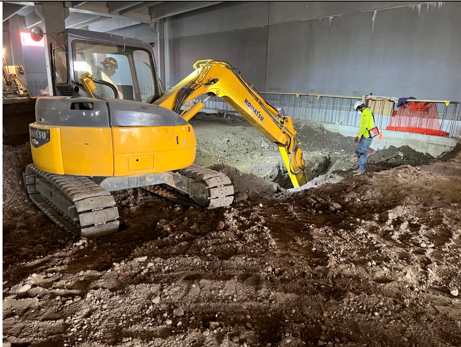
Photo 1: Looking north, Kingdom continues local storm drain trench excavation in grid B1.
