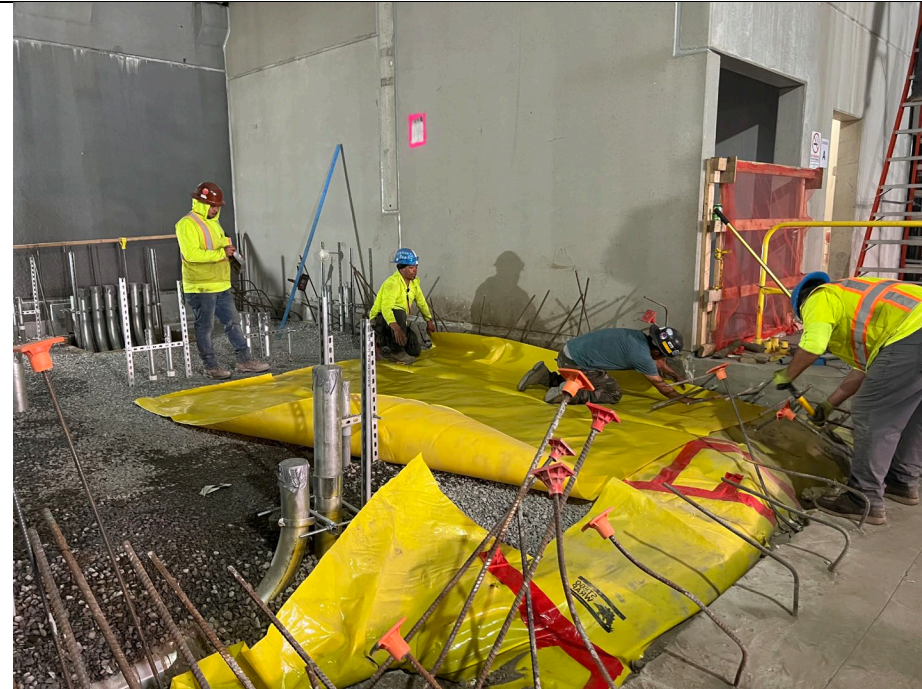
Photo 3: Looking east, view of Kingdom installing vapor barrier in grid A3 after backfilling.
