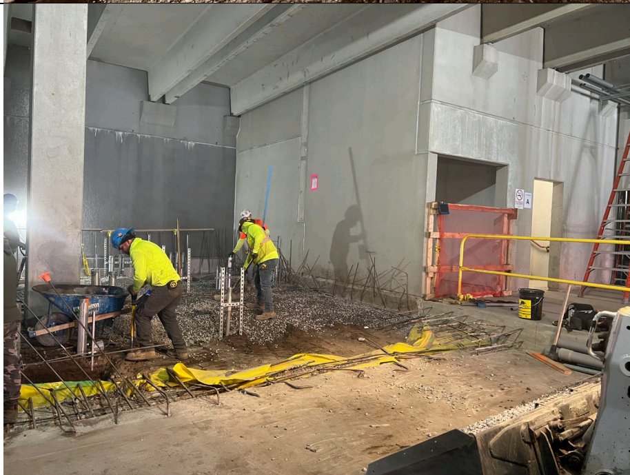
Photo 2: Looking east, view of kingdom backfilling portion of grid A3 with ¾" crushed stone.
