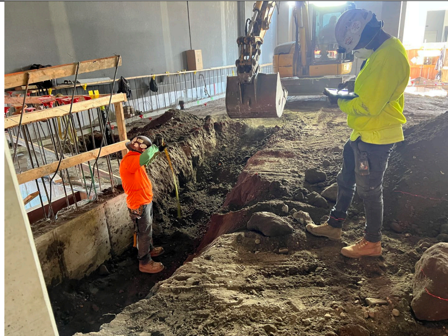
Photo 3: Looking northeast, Kingdom continues local storm drain trench excavation in grid A1.
