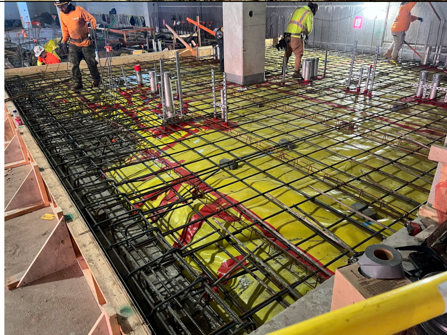
Photo 4: Looking northeast, view of Kingdom installing rebar in grid A3 in preparation for concrete pour.
