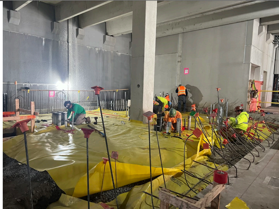
Photo 1: Looking southeast, view of Kingdom continuing vapor barrier installing in grid A3.
