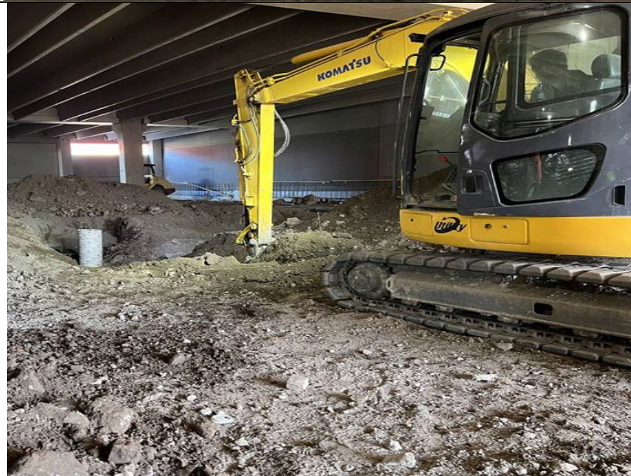
Photo 4: Kingdom performing minor excavation for trenching for additional utilities installation.
