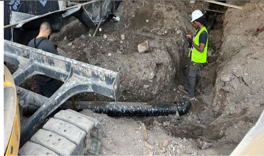
Photo 3: Looking west, view of storm drain installation connection.
