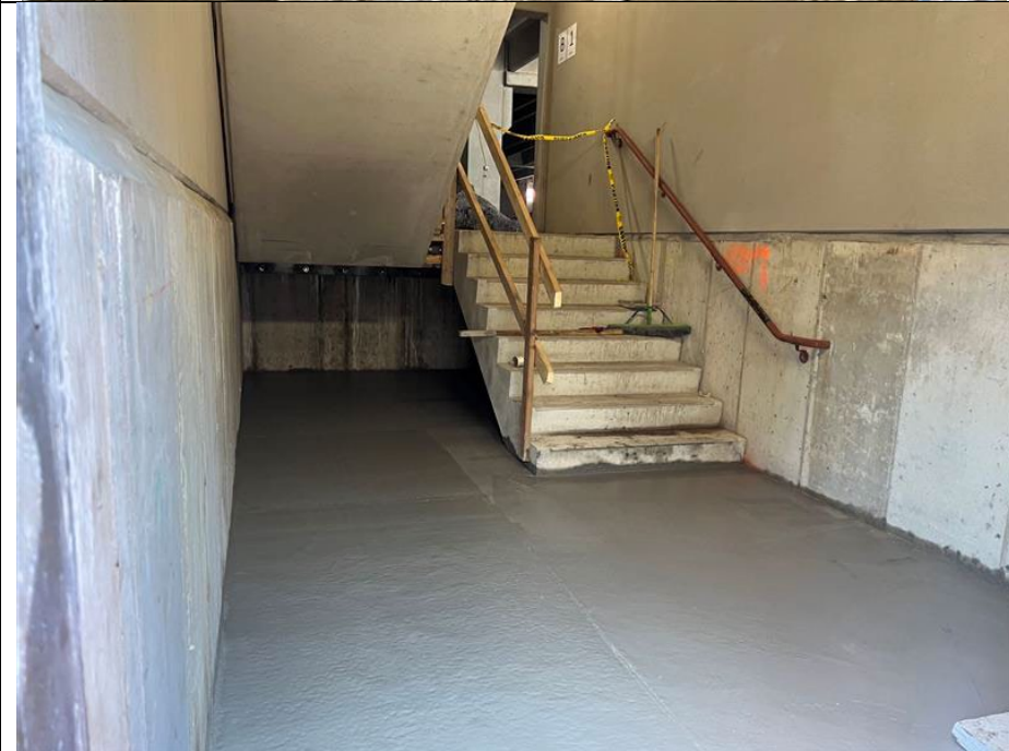
Photo 2: Looking west, view of finished pour in staircase B landing.
