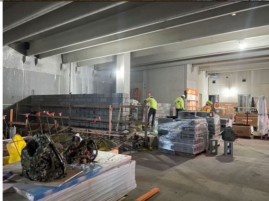
Photo 4: View of block going up for room in northeast corner of grid A3.
