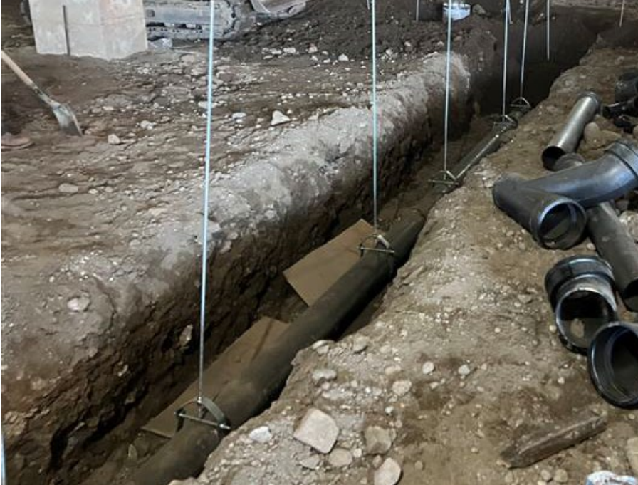
Photo 1: View of Kingdom installing storm drain trench in grid A2.
