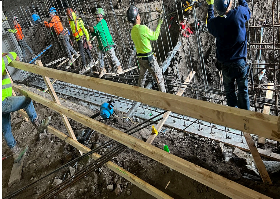
Photo 1: Looking northeast, view of kingdom installing rebar for additional wall.
