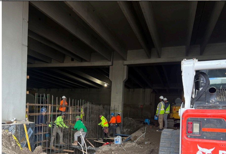
Photo 2: Looking south, view of Kingdom installing additional wall in A1.
