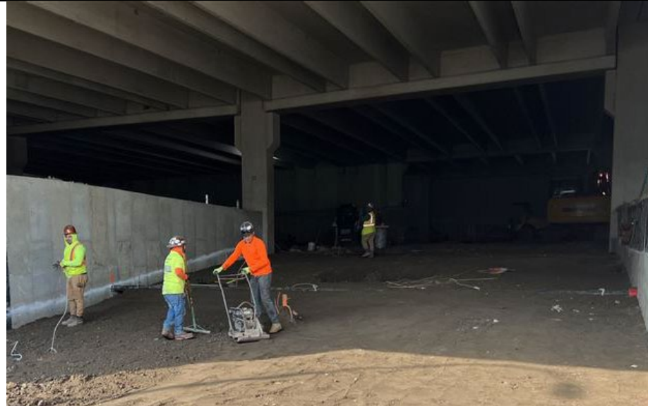
Photo 1: Looking northeast, Kingdom grading in grid A1 to form ramp.
