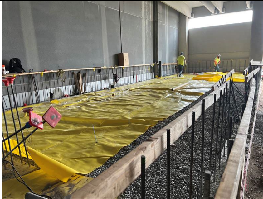
Photo 3: Looking northeast, Kingdom installing vapor barrier in north portion of grid A1.
