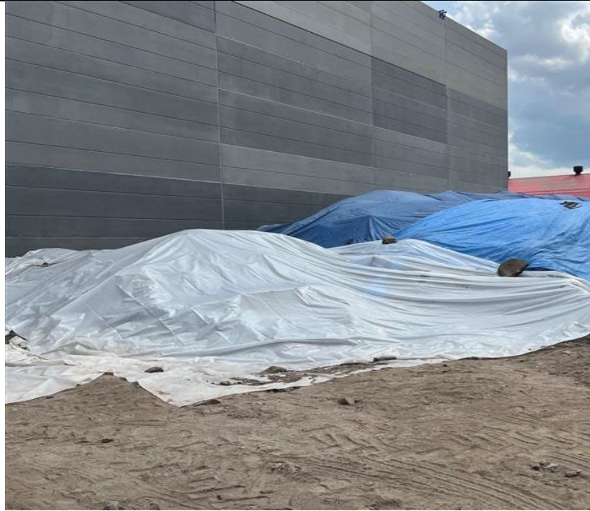
Photo 4: Temporary stockpile covered at the end of workday.
