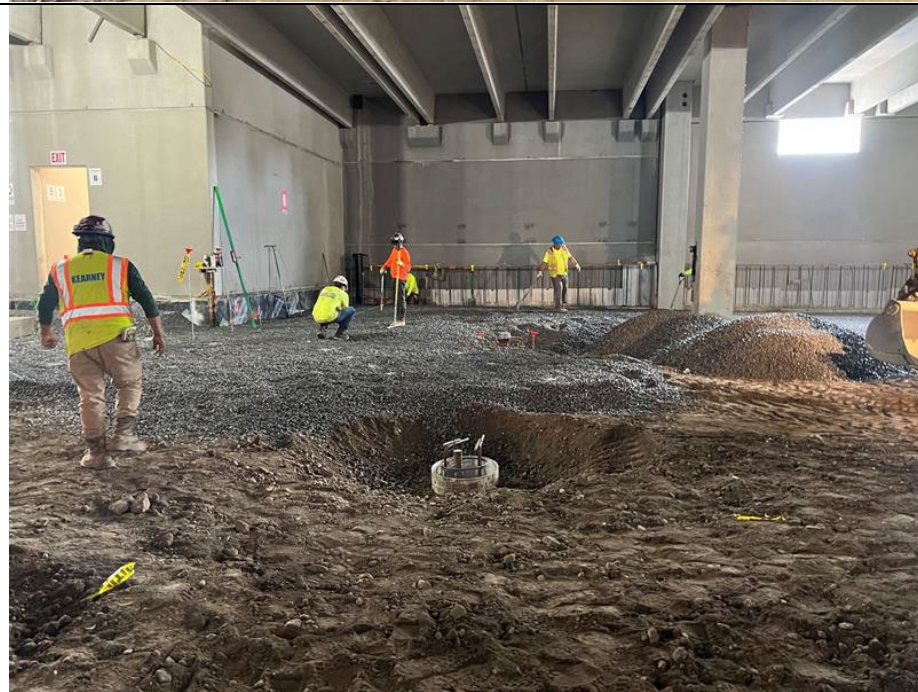
Photo 2: Looking east, kingdom backfilling grids A1 and A2 with ¾" stone.
