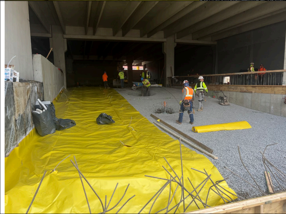
Photo 2: Looking west, view of ramp portion in grid A1 backfilled with 3/4" stone from Tilcon and vapor barrier installation.
