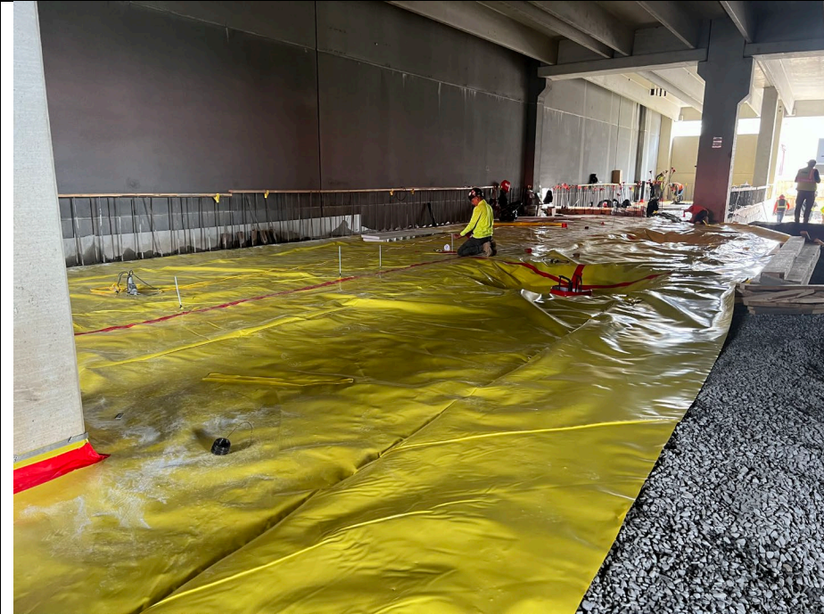
Photo 1: Looking northeast, progress of vapor barrier installation in grid B1.
