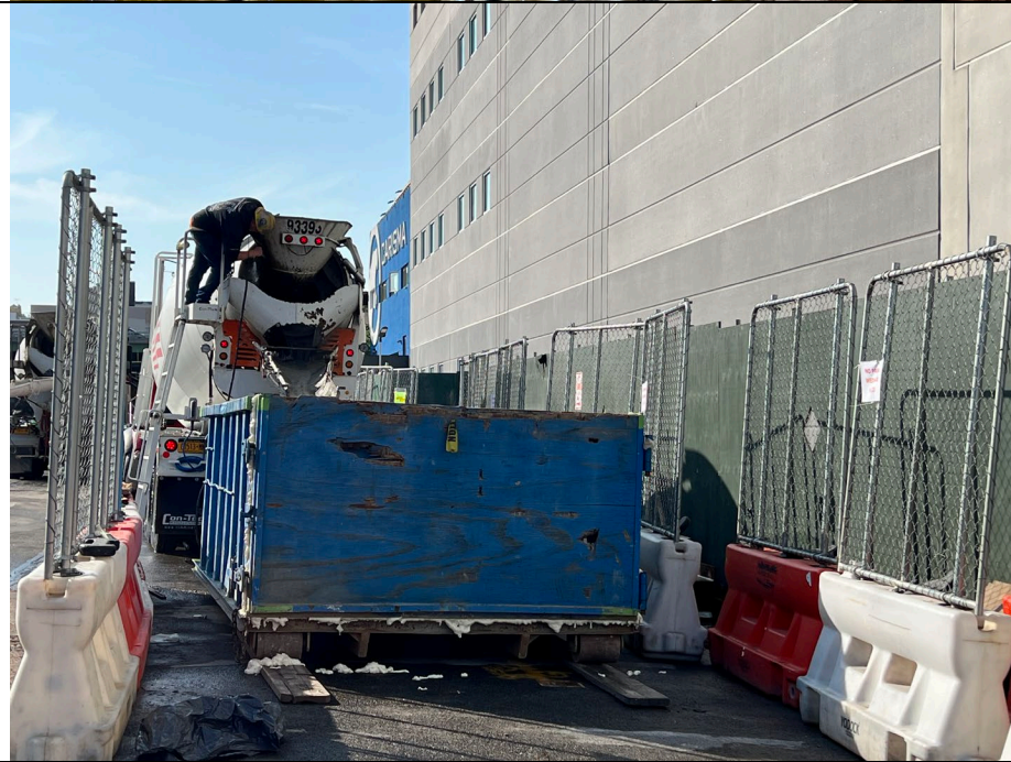
Photo 2: View of concrete truck driver using wash out box before leaving site.
