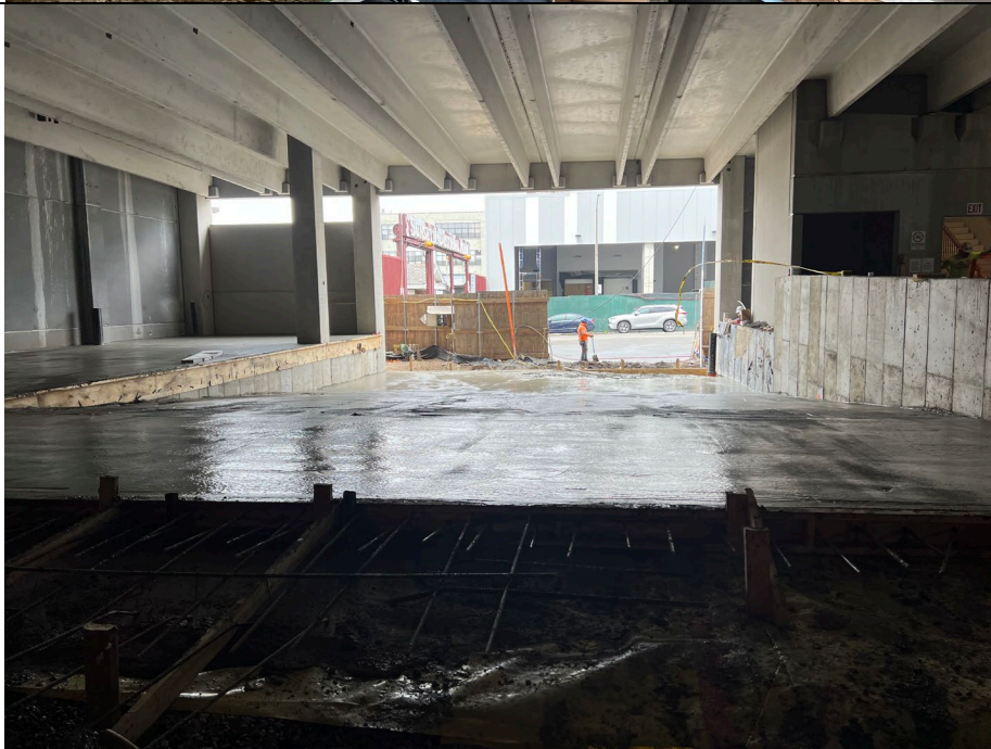
Photo 4: Looking east, view of finalized concrete pour for ramp in grid A1.
