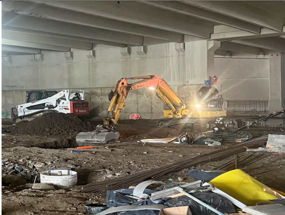
Photo 3: Looking west, Kingdom excavating in grid B1 for storm drain trench.
