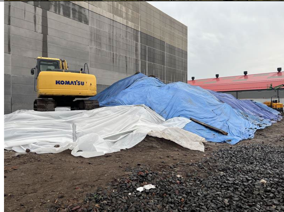
Photo 4: Status at the end of the work day; temporary stockpile was covered and secured.
