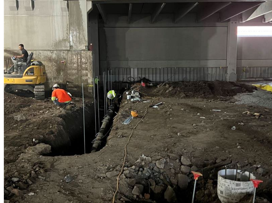
Photo 1: Looking west, storm drainpipe installation continues in grid B1.
