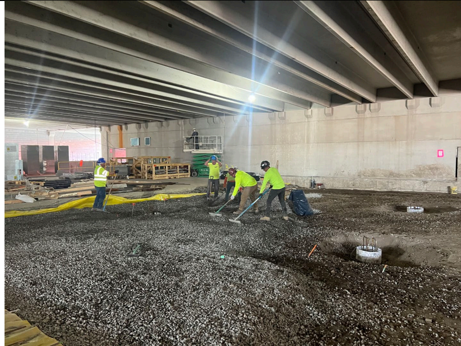
Photo 1: Looking southwest, Kingdom backfilling with ¾" stone from Tilcon in grid B2.
