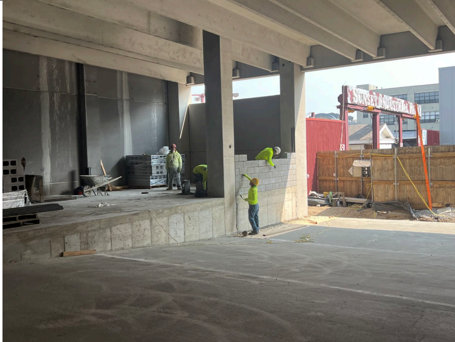
Photo 3: Looking northeast, block going up for room in northeast corner of grid A1.
