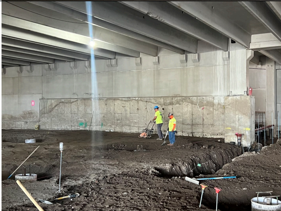
Photo 4: Looking south, Kingdom continues grading prior to stone installation.
